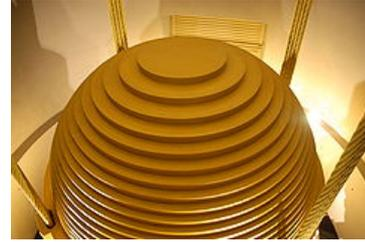
Figure 1.6: Tuned mass damped erected on Taipei101 skyscraper.
