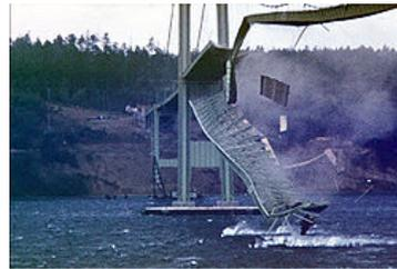
Figure 1.4: Tacoma narrows bridge collapse under 64 km/h winds.<sup>2</sup>
