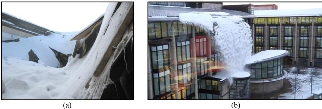
Figure 2. Examples of the damages caused by snow accumulation: (a) a collapsed roofs [3], (b) a massive snow fall from a roof in Scotland [4].
