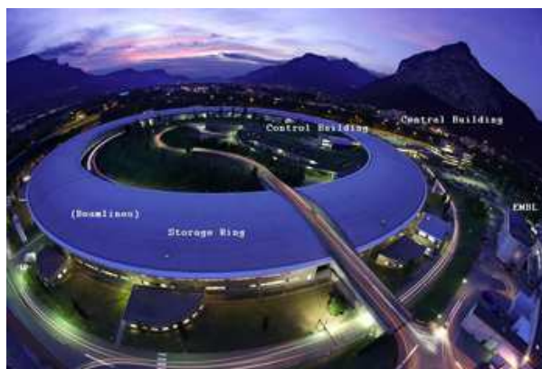
Figure 42 Photo de l'European Synchrotron Radiation Facility (ESRF).
