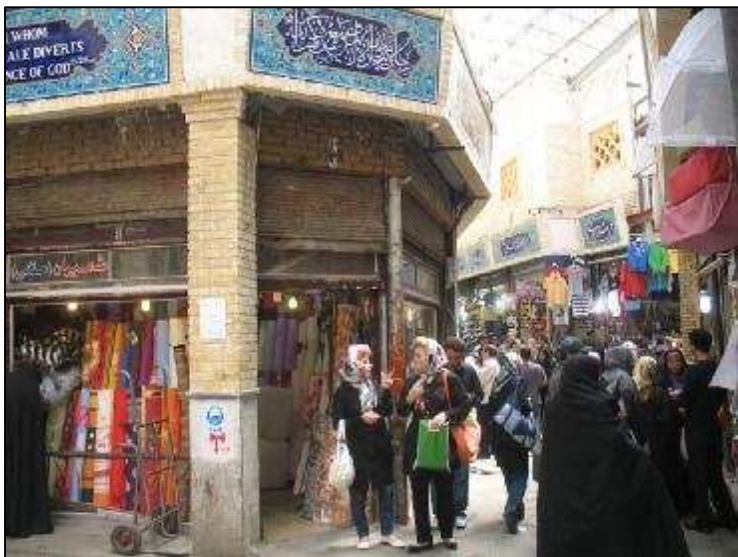
The columns and outside parts of the shops are reconstructed with brick and tile;
