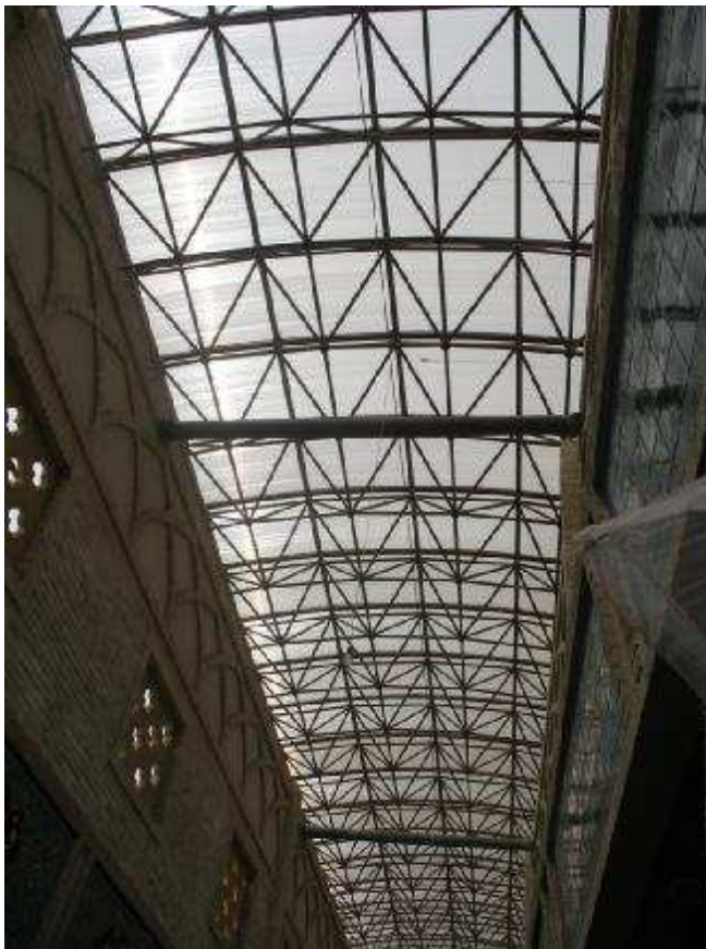
The new gable construction made shade and a safe space away from natural disasters also changing the overall atmosphere of the bazaar which was a wooden gable roof before the reconstructions
