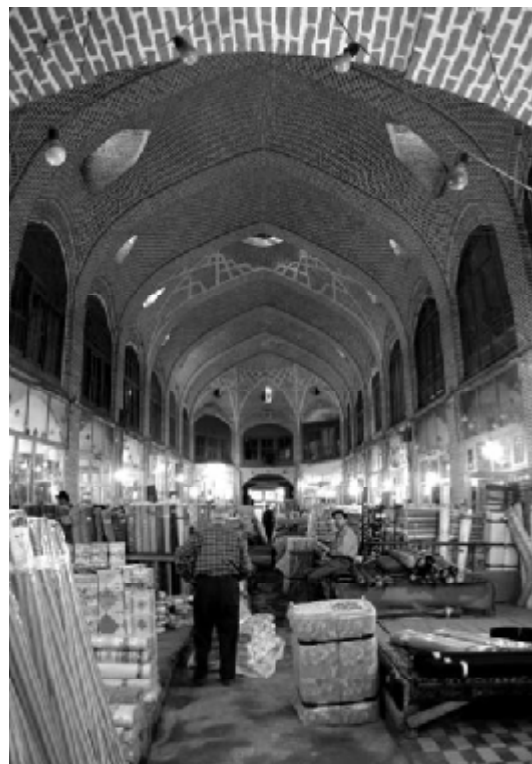
The main Raasteh(pathways) in the Tabriz traditional bazaar appear with domed ceilings, brick material and two storey shops located on its booth sides
