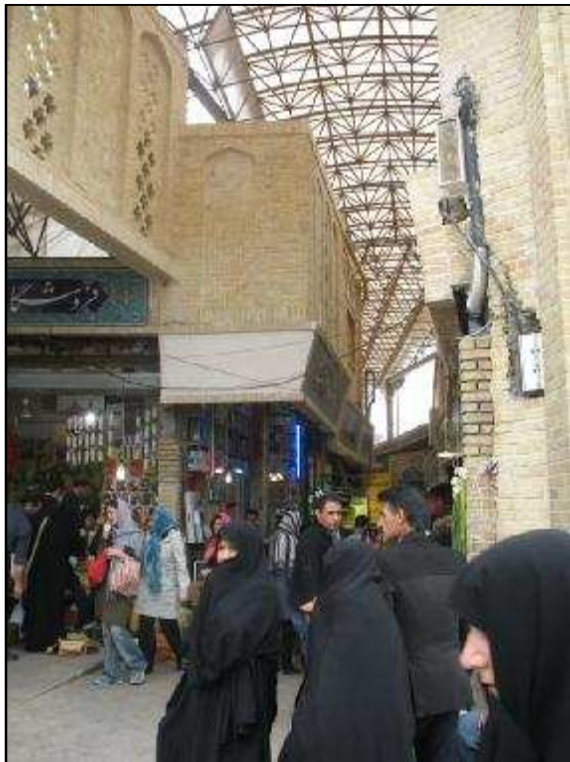
New reconstructions and materials in the Tajrish traditional bazaar roof
