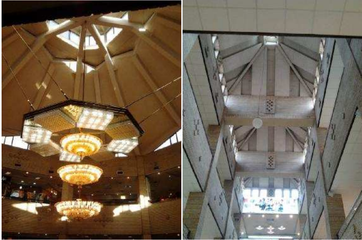
The ceiling situated on top of the water basin in the Golestan shopping center is a repetition of the polygon on surface Glass windows lead light indirectly inside plus a great chandelier is hanging from the ceiling for extra artificial light
