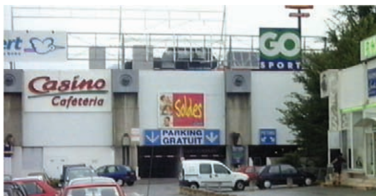
Figure 26 : Façade de Grand'Place Grenoble. Parking Nord
