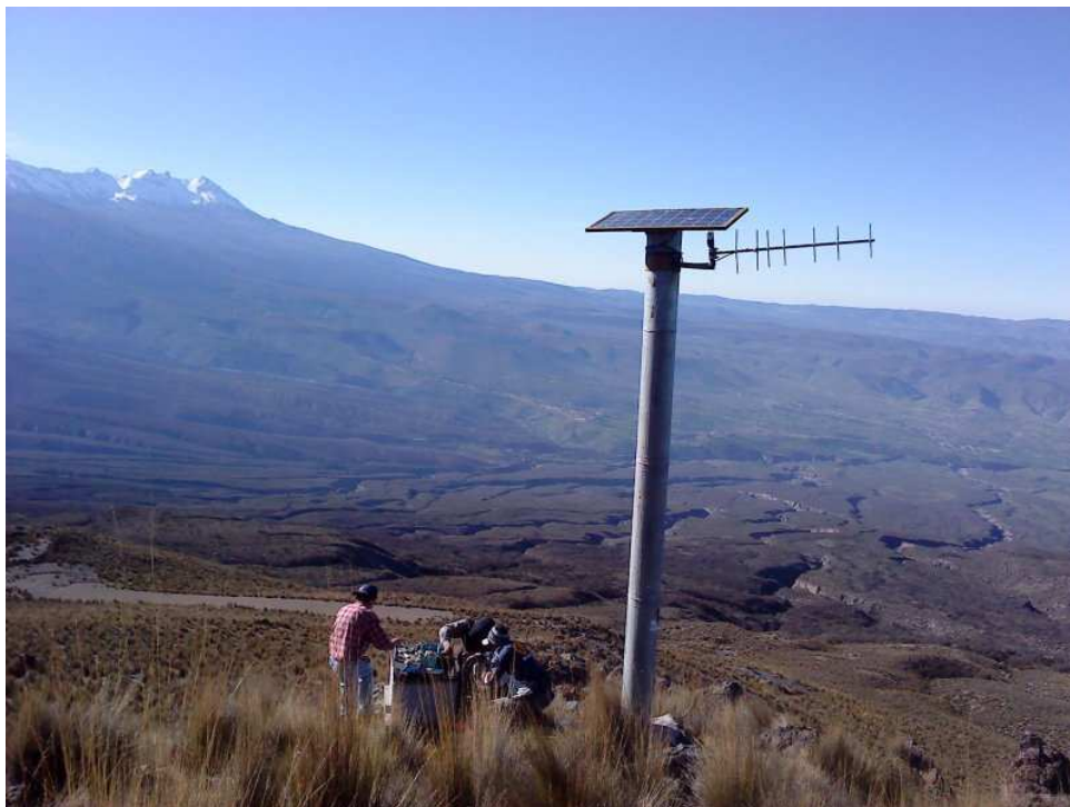
Figure 1.31: A view of a seismic station used to send data to the observatory, at the top of the pole a Yagi antenna and a solar panel can be seen
