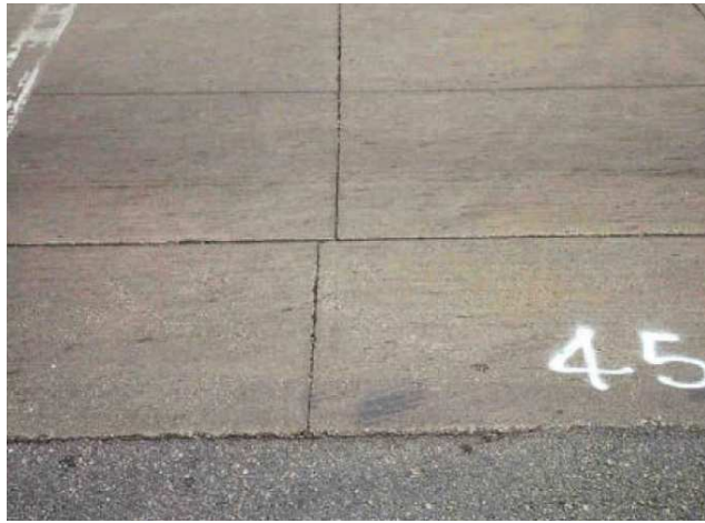
FIGURE 1.21 – Mouvement de panels [Kim et al., 2009]
