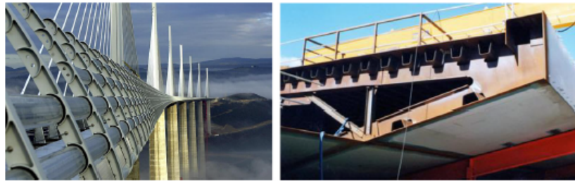
FIG. 1—View of the Millau Viaduct (France)—the highest bridge and the longest multiple cable-stayed bridge in the world.
