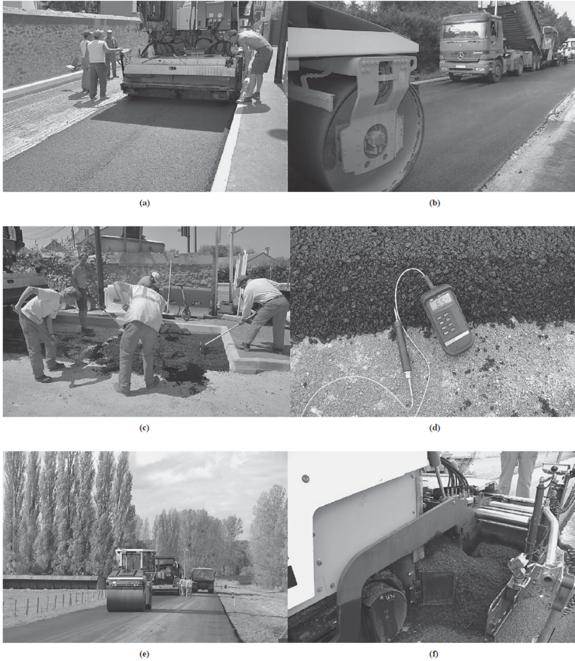
FIGURE 8 Placing LEA mixture produced by industrial plant.
