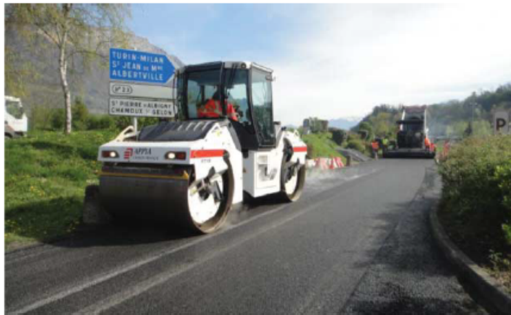
Figure 17. GB5 0/14 mm with Budillon aggregate and SBS modified binder Biprène 41 (proprietary composition) and 15% RAP near Chambéry. In-place density: 97%; modulus E^* (15°C–10 Hz): 15,900 MPa.
