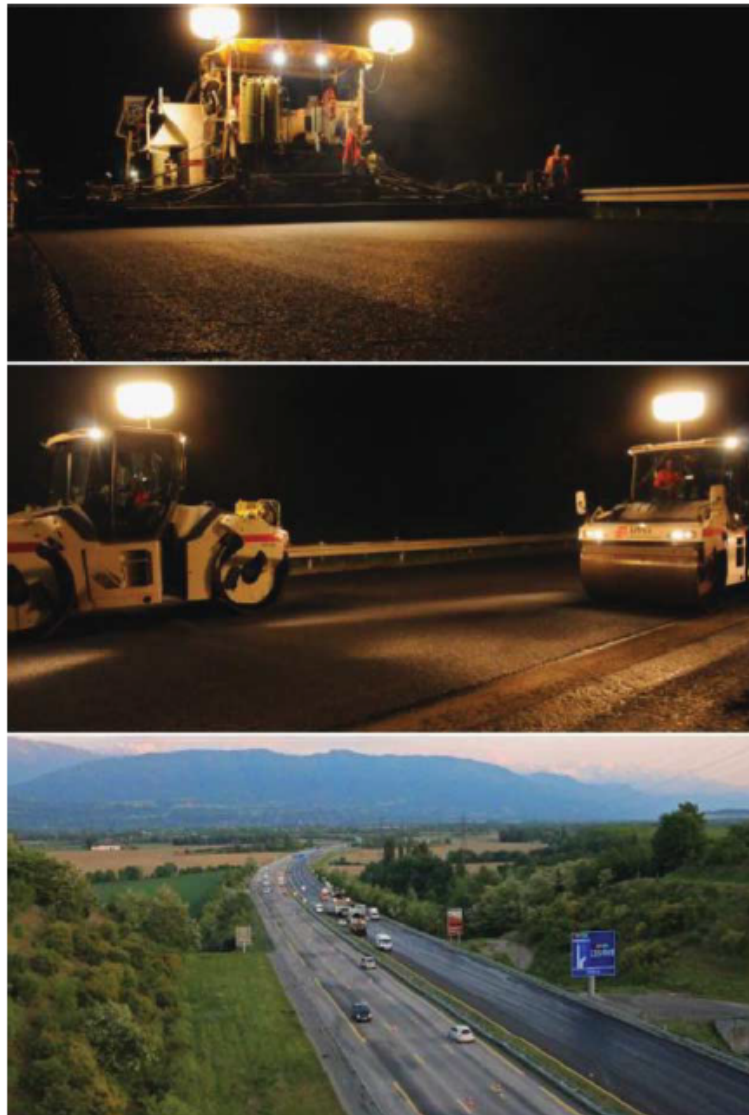
Figure 18. 12,000-ton GB5 0/14 roadwork on the French A43 toll highway (AREA network, Chignin-Francin section) in the alpine area. Budillon aggregate, 15% RAP (reclaimed asphalt pavement) and PMB's Biprene 41 & Orthoprene were used.
