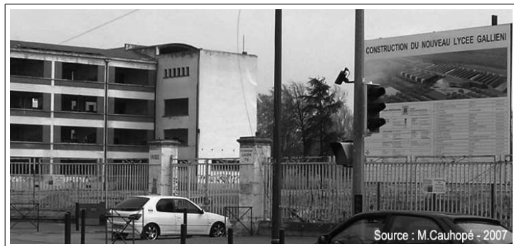
Figure 10: Reconstruction du lycée Gallieni (2007)
