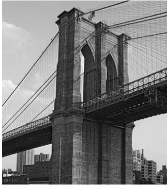
Figure 1.3. Brooklyn bridge – New York 1883
