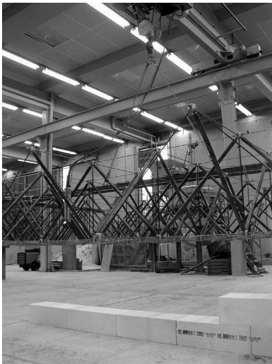
Figure 2.25. Tensarch en construction
