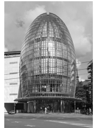
Fig. 10a Renzo Piano Building Workshop, Peek and Cloppenburg, Colonia (2007)
