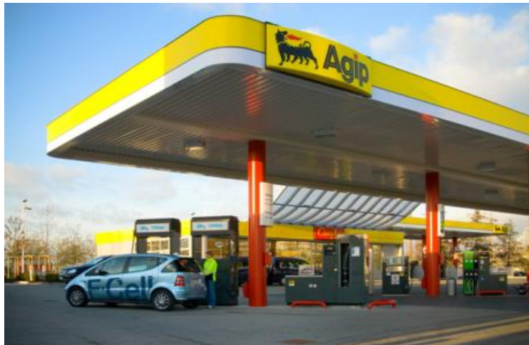
Figure I-4: Frankfurt hydrogen filling station, available as a bi-product from a chlorine electrolysis plant and transported via a high pressure 1.7 km long transport line to the fuelling service station [19].
