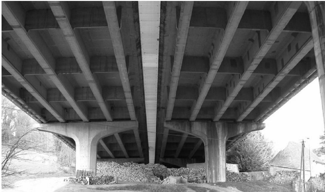
Figure 3.2: View of the instrumented Roberval Bridge
