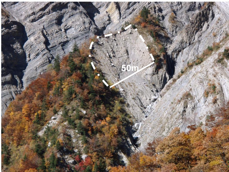
**Figure 33** View of a landslide ( $26\,000\text{ m}^3$ ) in the upper catchment of the Manival which failed in the winter of 1991; during the summer of the same year, two channel-debris flows deposited a sum of  $25\,000\text{ m}^3$  in the sediment trap
