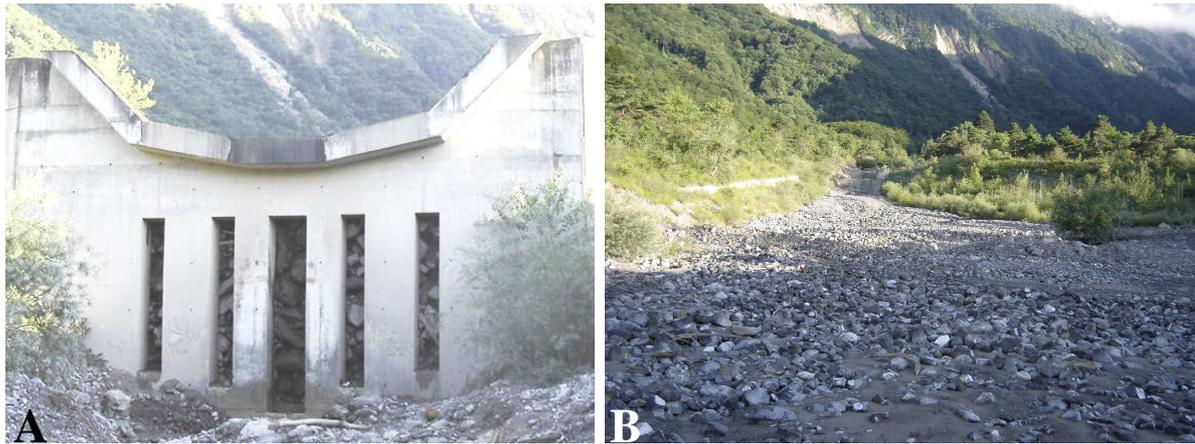
**Figure 20** View of the sediment trap after a debris-flow with (A) the dam blocked by the boulder front with tree debris and (B) the rest of the trap filled with finer sediment.
