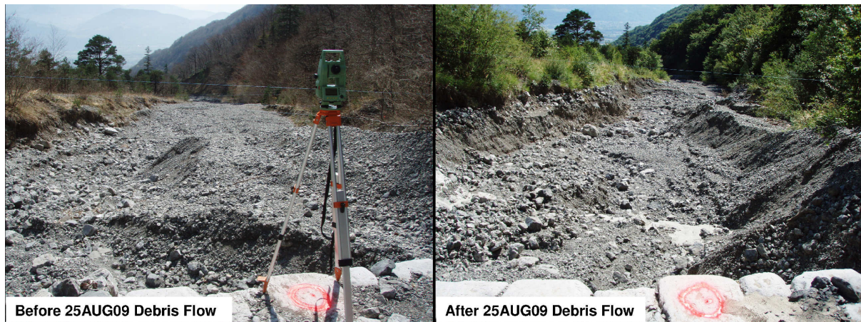
Figure 26 Photo sequence displaying channel scouring of the August 2009 debris-flow in the main channel of the Manival; views looking downstream
