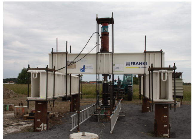
Figure 3: Two-way pile load test set up at Merville
