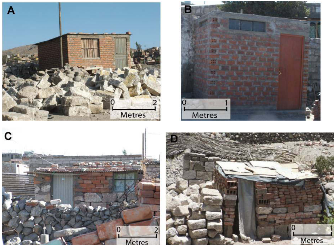
Figure 4.12: Unconfined masonry dwellings in Arequipa. Dwellings A and B are constructed of red clay brick with mortar, whereas dwellings C and D are constructed from a mixture of ignimbrite and red clay brick with no mortar.
