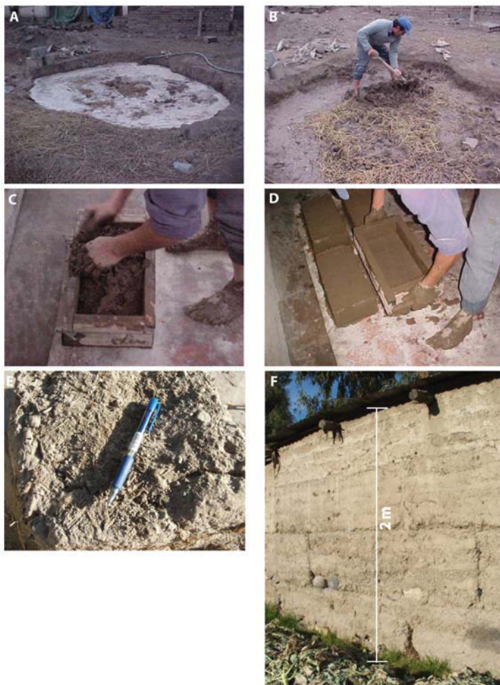
Figure 4.15: Making adobe bricks – A: a big pit is made and water added to make the ‘mud’, mud is then scooped up ( B ) and put into moulds ( C ), bricks are then turned out ( D ) and left to dry (photos obtained from Victor Rodriguez). E: An adobe brick from Arequipa – note the muddy texture with bits of straw. F: An adobe dwelling on the lower terrace side of the western side of the Río Chili in the city centre.
