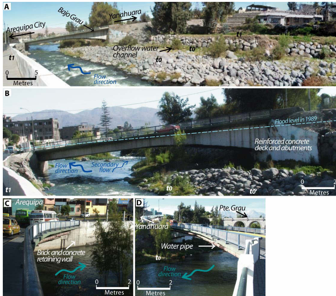
Figure 4.41: A: Puente Bajo Grau, a one-way bridge connecting the Yanahuara district on the western side of the Río Chili River with the city centre. Note the different terraces on the western channel edge. B: Downstream view of Bajo Grau showing the slope of the bridge deck to the east. C: Curvature of the bridge to the south directing one-way traffic onto Avenue de la Marina. D: View of the bridge westwards towards Yanahuara, face-on to traffic, and Pte. Grau in the background. Note the pipe running under the bridge deck.
