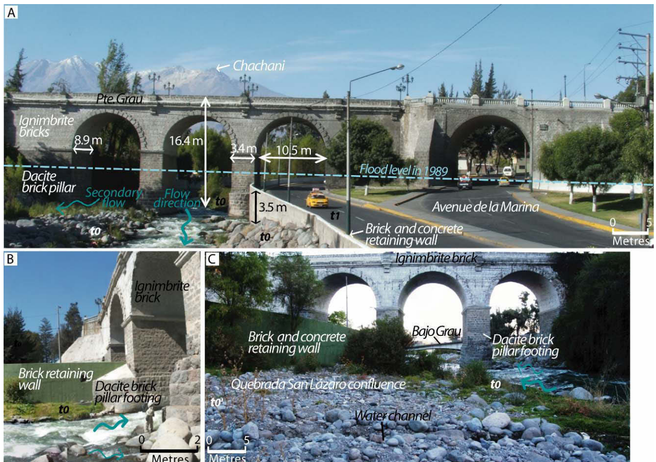
Figure 4.40: The iconic colonial-style ignimbrite masonry multiple span arch bridge ‘Puente Grau’. Note the gradient of the road sloping away from the river. A: Downstream view of the bridge crossing the Río Chili. B: Upstream view of the large pillars and footings constructed from dacite lava masonry from the western side of the river. C: The upstream view of the bridge, from the eastern side, at the confluence with Quebrada San Lázaro.
