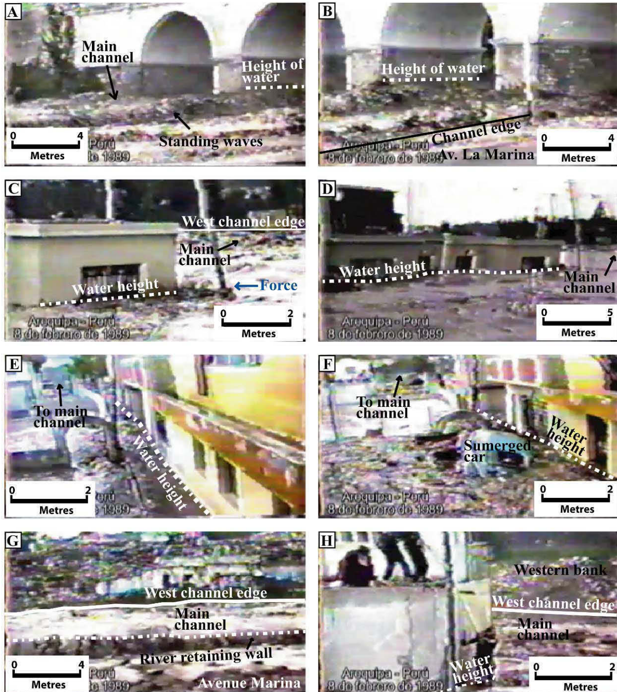
Figure 2.7: Frames taken from film footage showing the events and damage caused by the 8-9 February 1989 flood in Arequipa. A and B: Flow in and around the Puente Grau Bridge in the centre of the city. C and D: the flow height around a house on the eastern side of the Rio Chili, downstream of the Puente Grau Bridge. E and F: An increase in flow depth can be observed between the two snapshots. A car has also been carried away by the flow. G and H: the flow within the Rio Chili channel can be observed. The height of the flow is above the retaining walls which are usually 3.5 m above normal flow. The effects of the flow on buildings can also be observed in snapshot H. Snapshots are obtained from unedited film from the local regional TV channel (Channel 8) viewed on “Youtube”.
