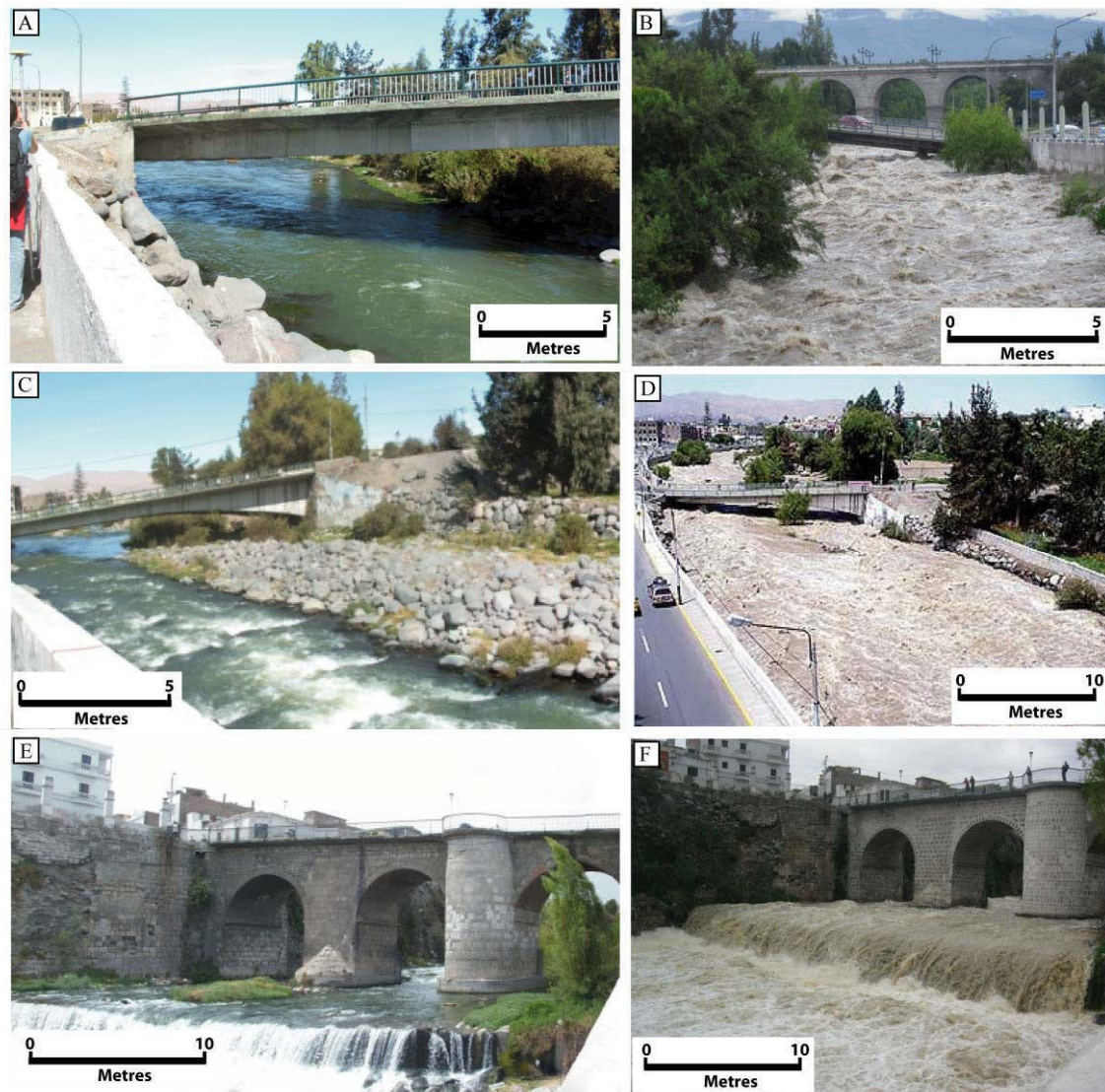
Figure 2.14: Before and after photographs of the flooding in the Rio Chili – before photos are taken in 2007 and 2008, and after photos were taken on 23 February 2011 (obtained from GrupoRPP www.rpp.com.pe ). A and C show the channel and bridge height of Puente Grau during normal river flow while B and D show the height of the flow (just under the bridge deck) and absence of terraces as can be viewed in C. E and F are downstream of Puente Bolognesi, again the absence of islands can be noted in F. Also the level of the river is noticeably higher in F than E.
