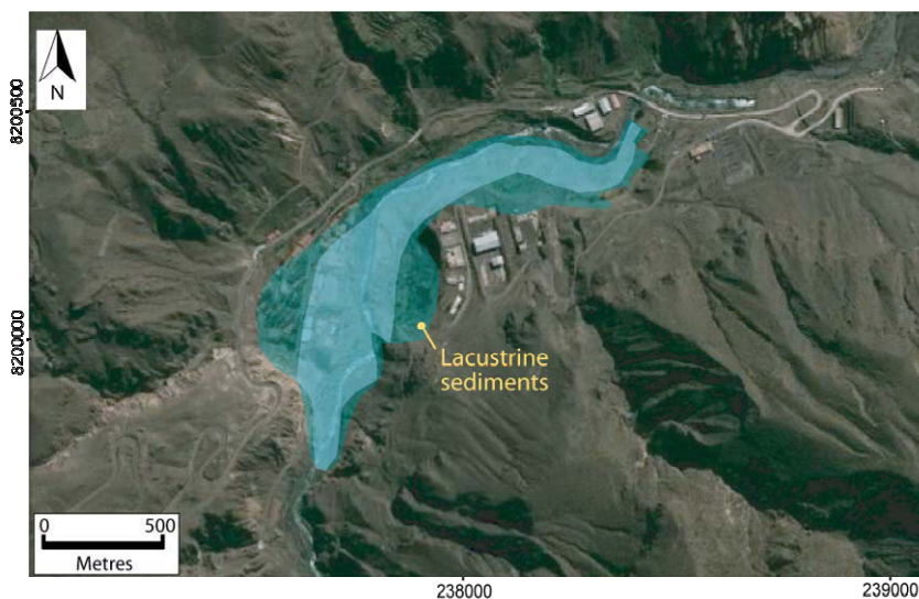
Figure 2.17: area where a lake could form in the upper Rio Chili canyon (near Charcani V). The lighter blue represents the likely area where a smaller lake would form, the darker blue representing the likely area flooded by a moderate sized lake. Image from Google Earth.
