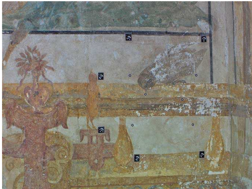
Figure 1.3: Flaking wall painting representing a bird on a balcony. Coded and uncoded targets are scattered around the area of interest.
