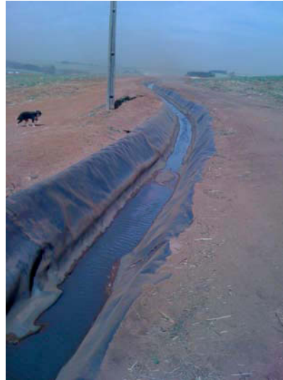
Figure 5 - Coated channel at Usina Catanduva (Catanduva, São Paulo, Brazil) following the new legislation.
