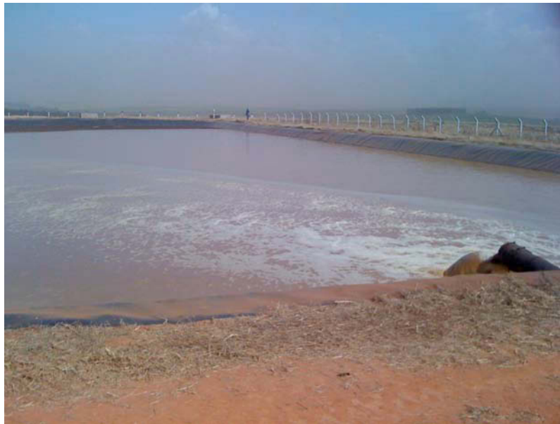
Figure 3 – Depuration LPB AH2on where vinasse is stored at Usina Catanduva (Catanduva, São Paulo, Brazil). At the day this picture was taken, the flow of vinasse was 350\text{m}^3\cdot\text{h}^{-1} .
