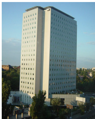
Figure 2.14: BRD instrumented building – headquarters of BRD – Société Générale Bank in Romania.
