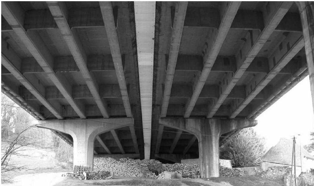
Figure 3.2: View of the tested girder bridge
