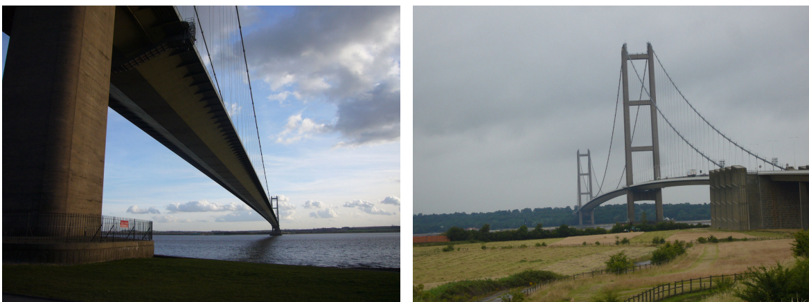
Figure 8.11 – Views of Humber Bridge from north and south.
