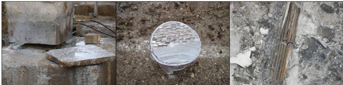
Figure 9.3 – Destructive damaging; a) cutting through one of the columns, b) and c) successive intersecting of prestressing tendons [VCE09].
