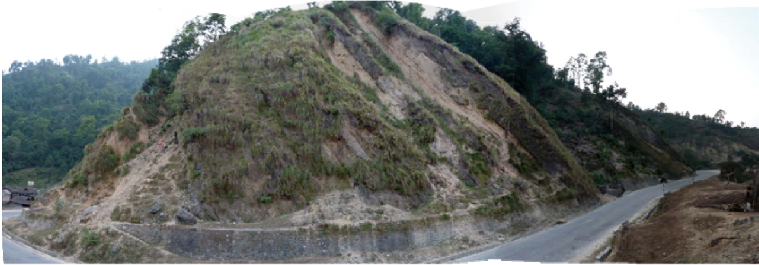
FIG 3 - Pictures from the Surai section.
