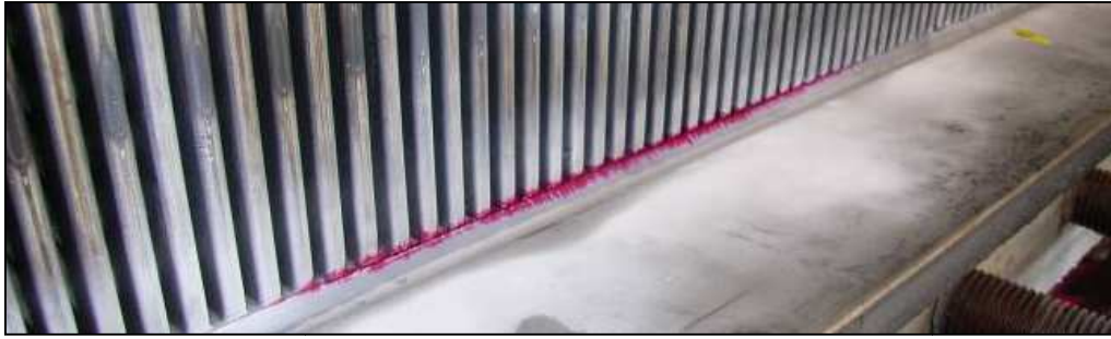
Figure I.11 - Failure along the column liner
