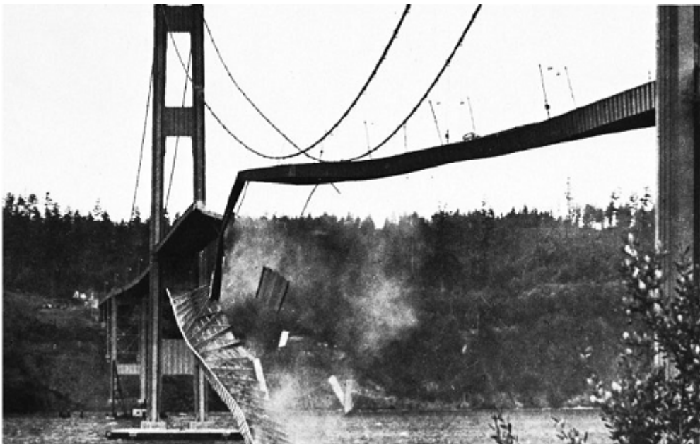
Figure 1.2. Tacoma Narrows bridge collapse under wind-induced vibration [1].
