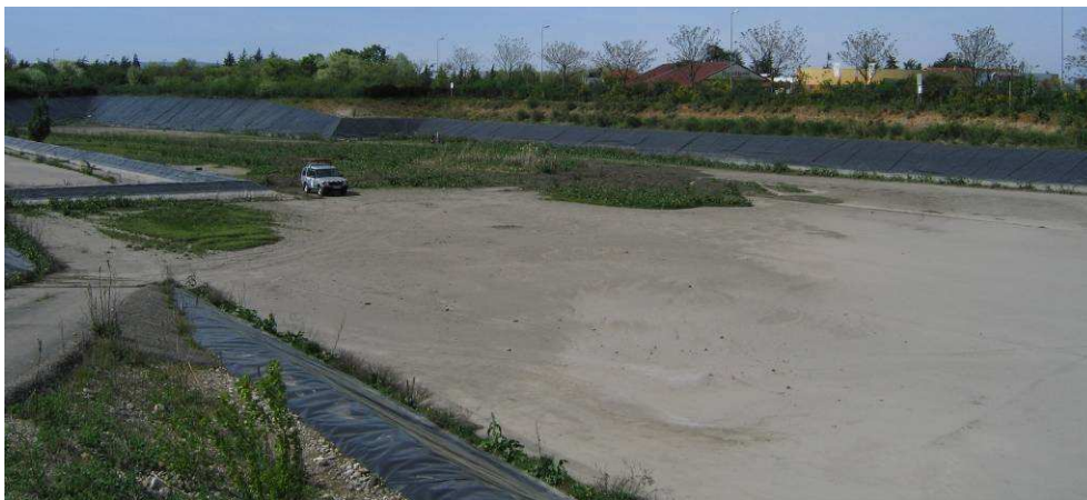
Figure 4-1 Accumulated sediment in the Django Reinhardt basin on 14/04/2011
