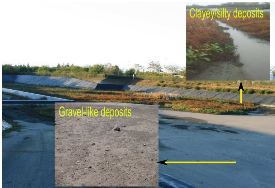
Figure 4-6 Pictures of gravel-like sediment and of clayey/silty deposits accumulated in the Django Reinhardt basin. The picture of gravel sediment was taken in 2011 and the picture of clayey /silty deposits was taken in 2012.
