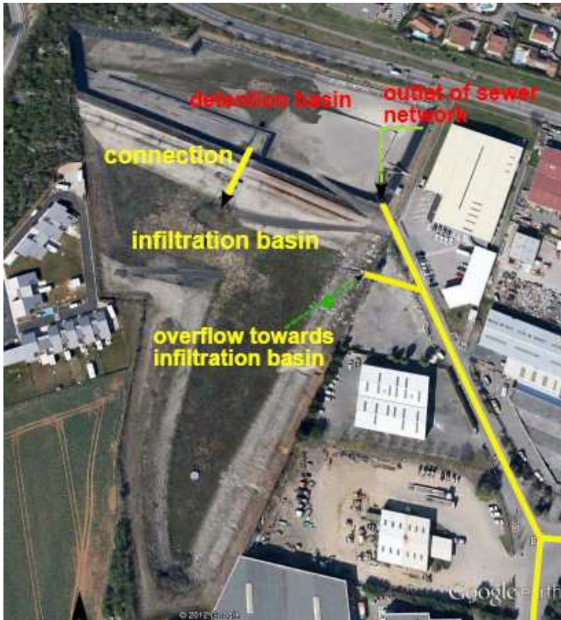
Figure 3-3 View of Django Reinhardt detention-settling and infiltration facility (photo of 15/03/2012 from Google map)
