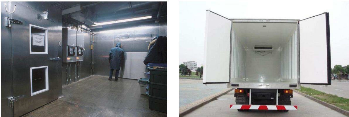
Figure 4.36: On the left hand side: example of a cold storage room. On the right hand side: example of a refrigerated truck.
