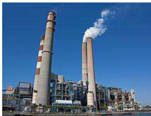
Figure 4.45: Example of power plant.
