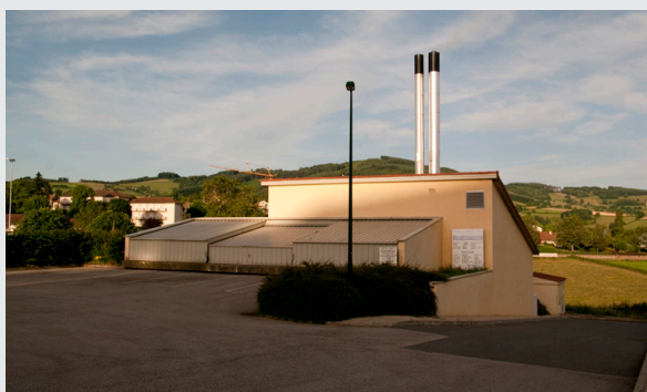
Fig.173 Chaufferie bois de Tramayes (CHAMODOT, 2012)
