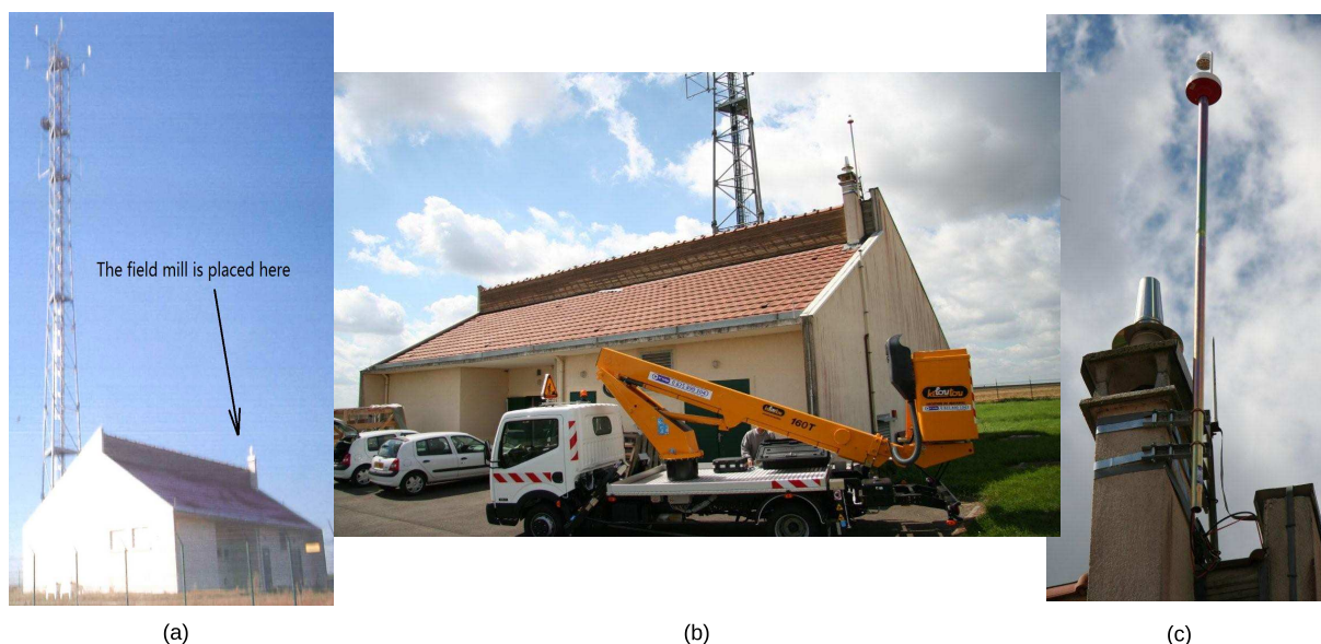
Figure 1.11: Position of the field mill: (a) general view; (b) ground station building; (c) field mill above the chimney.
