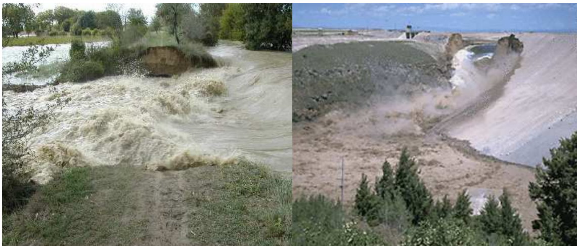
Figure 1.1. Breach caused by flooding of the Virdourle river in 2002 (left) and breach of the Teton Dam, 1976 (right).
