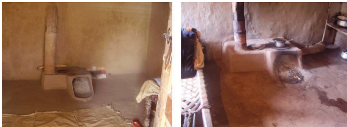
Figure 7.6 — Inside kitchens built in the rooms. Source : S. Abidi.
