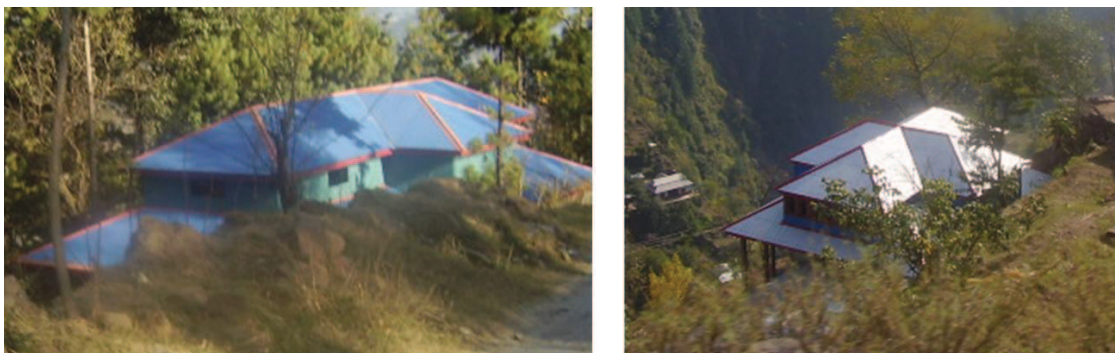
Figure 6.36 — Houses with hip and valley roof on tower roof. Source : S. Abidi
