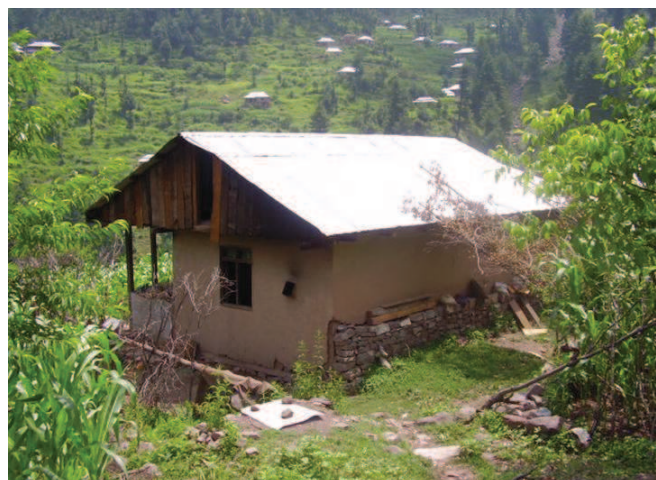
Figure 6.29 — An example of attic having gable roof. Source : S. Abidi
