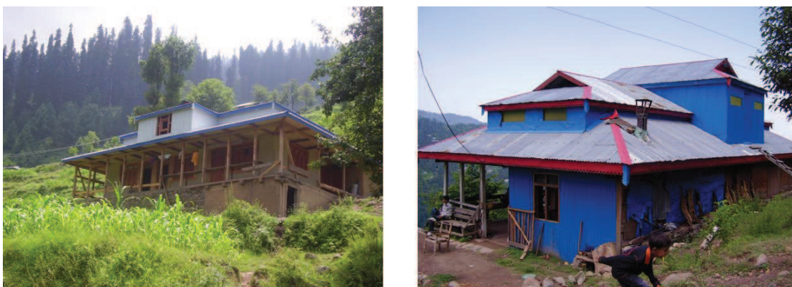
Figure 6.40 — Dutch gable roof on independent structure. Source : S. Abidi
