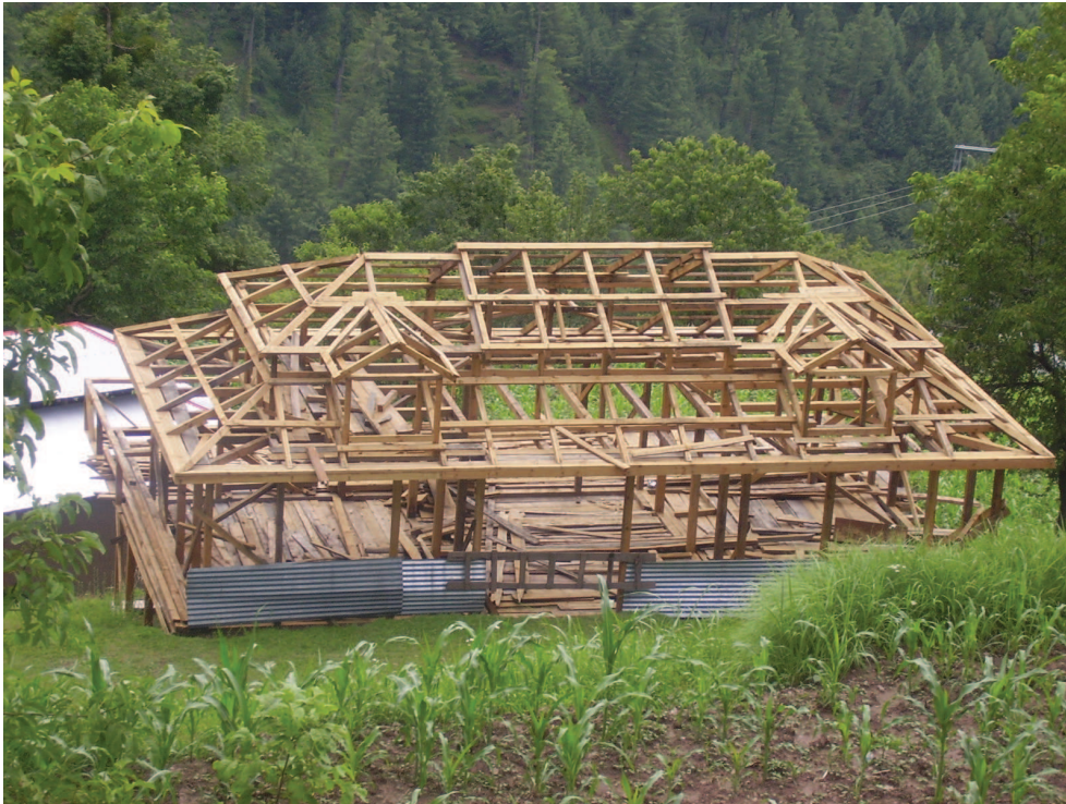
Figure 6.2 — Tower roof is under construction. Source : S. Abidi
