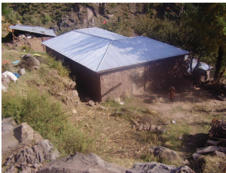
Figure 6.52 — A reconstructed single storey house truly following erra’s guidelines. source : S. Abidi
