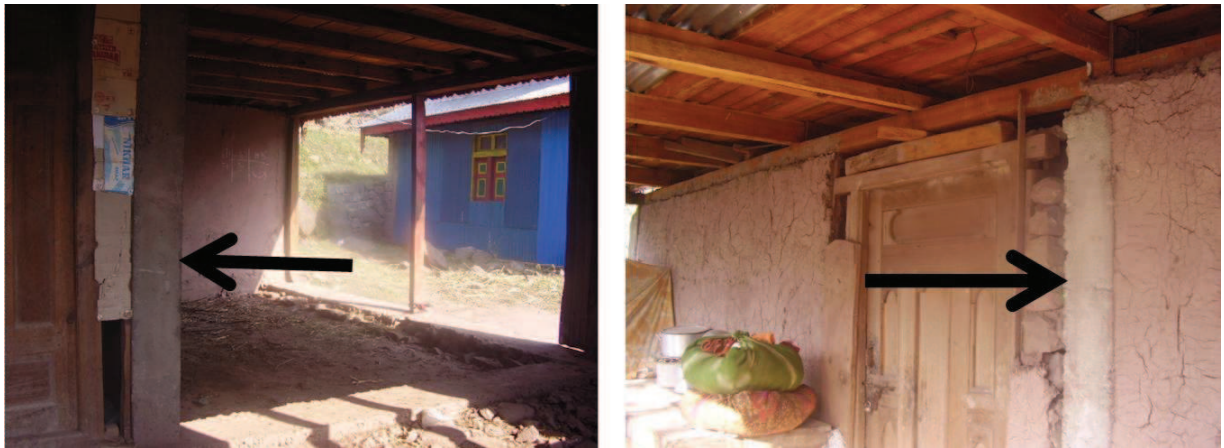
Figure 7.32 — Presence of concrete columns in dhajji houses. Source : S. Abidi.
