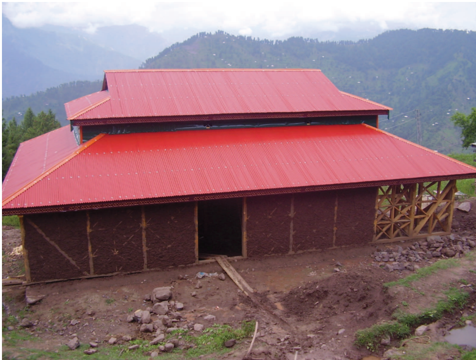
Figure 6.1 — A type of tower roof. Source : S. Abidi
