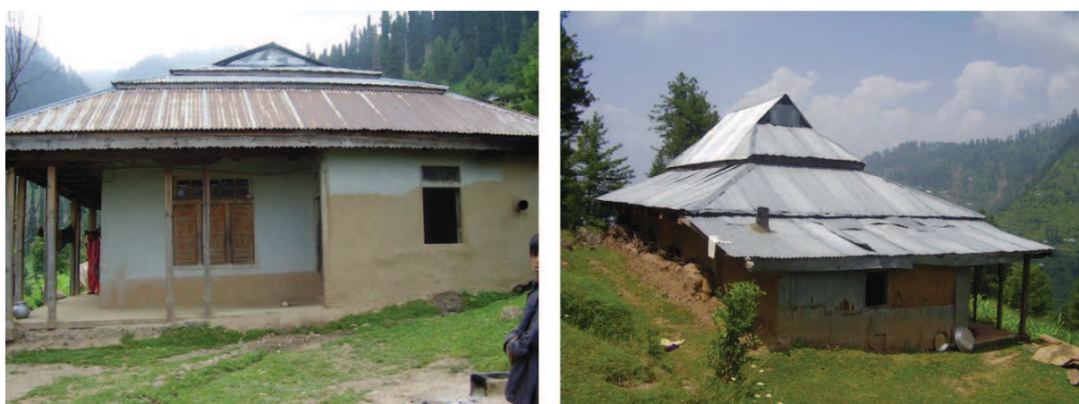
Figure 6.45 — CGI Sheets make the cladding for attic. Source : S. Abidi
