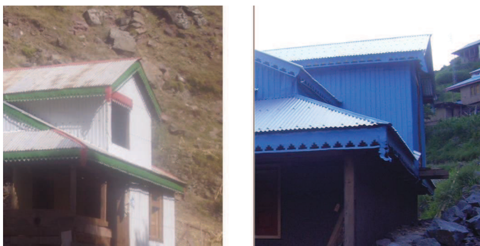
Figure 6.41 — A space formed on the roof and is independent of the main structure while it has gable roof on its top. Source : S. Abidi
