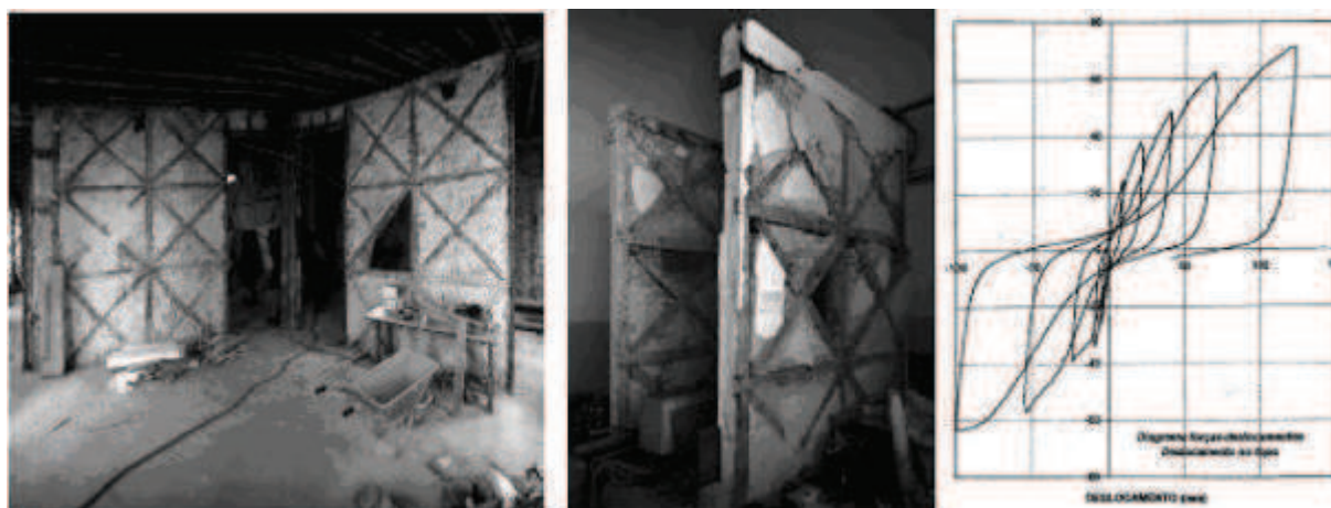
Figure 5.15 — Left : 18th Century building in central Lisbon showing "Pombalino gaiola" construction, 2003. Centre : Gaiola wall sections from a late 18th or early 19th C. building after having been tested. Right : Hysteresis diagram from one of the wall tests of the walls in both left figures ([Langenbach, 2007])
