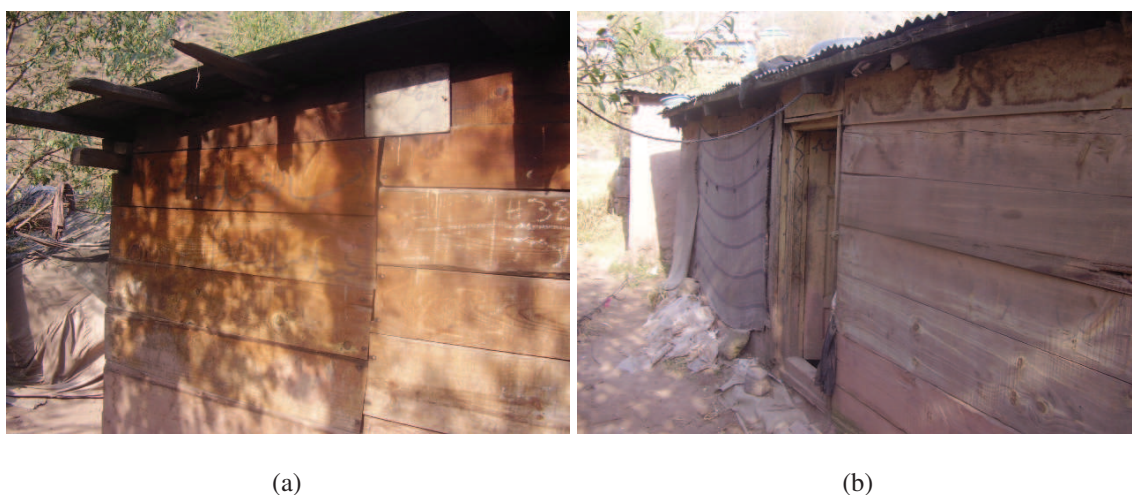
Figure 5.30 — Wooden planks are nailed on dhajji walls. source : S. Abidi
