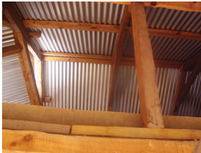
Figure 6.74 — A view of tower roof frame from the ground floor. no diagonal elements are observed. Source : S. Abidi
