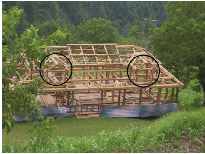
Figure 6.42 — Under-construction house having dormers. Source : S. Abidi
