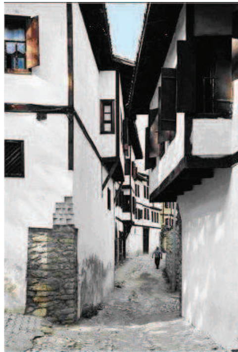
Figure 5.10 — The upper story is almost always constructed with himis. ([Langenbach, 2003])
