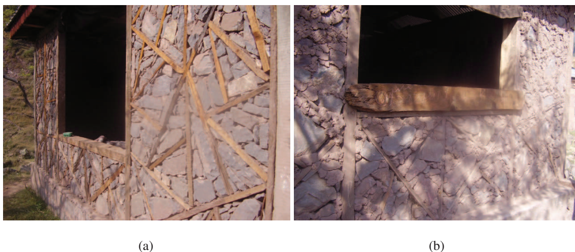
Figure 5.26 — Exposed dhajji walls. Source : S. Abidi.
