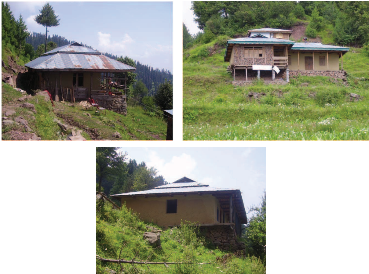
Figure 6.83 — People have built on hazardous sites. Source : S. Abidi.
