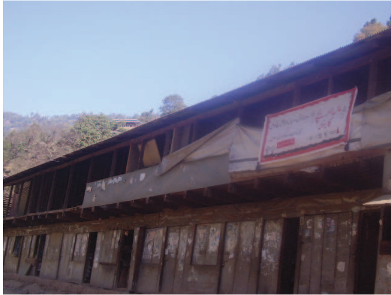
Figure 5.17 — Front elevation of Qadri market. Source : S. Abidi
