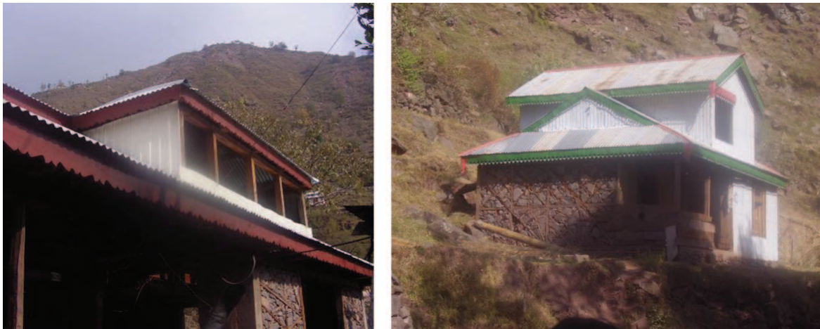
Figure 6.46 — Tower roof houses showing dhajji dewari on ground floor. the upper structure is covered with CGI sheets and is distinctly framed out of ground floor. Source : S. Abidi
