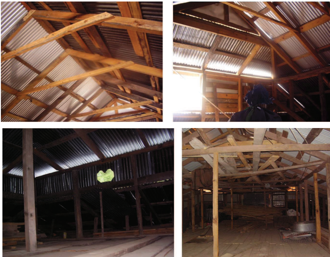
Figure 6.71 — Rafters and purlins in timber frame. source : S. Abidi
