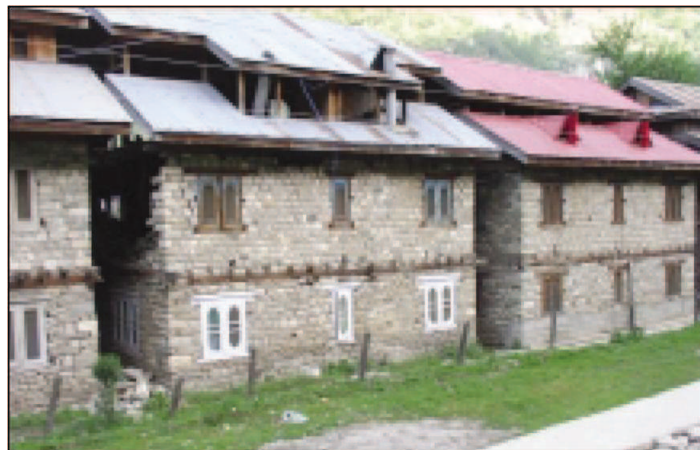
Figure 6.62 — Attic in urban buildings of Kashmir. Source : [UNDP and UNESCO, 2007]
