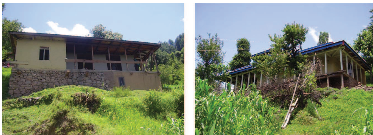
Figure 7.24 — Issues of the sight in reconstructed houses. Source : S. Abidi
