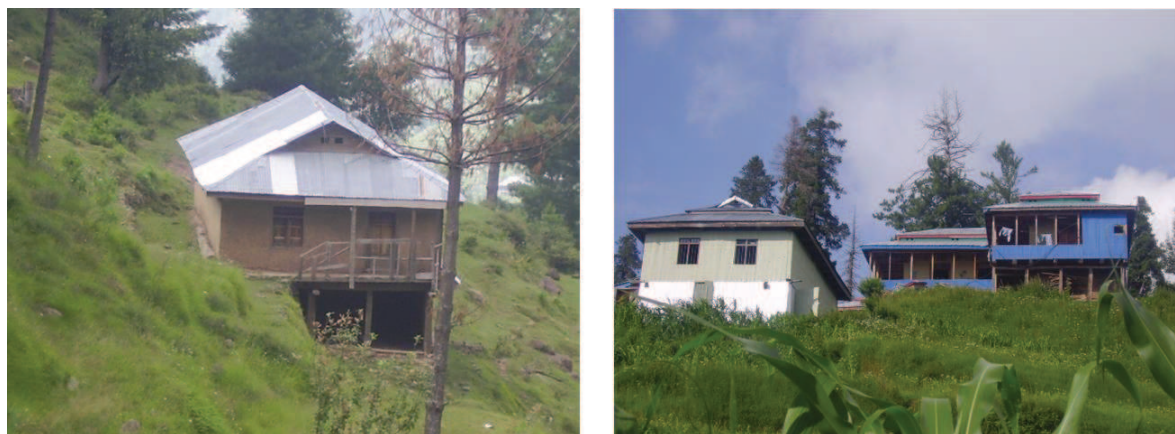
Figure 8.29 — Soft storey houses found in AJK. Source : S. Abidi
