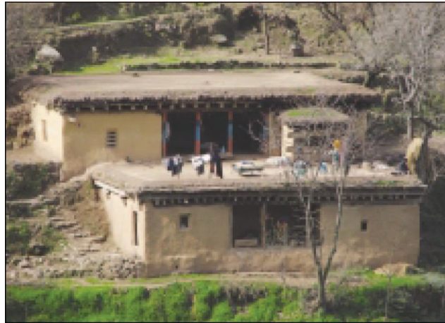
Figure 6.7 — Terraced house present before earthquake. Source : [UNDP and UNESCO, 2007]
