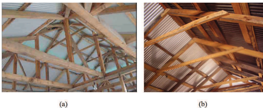
Figure 6.44 — Frame of tower roof. (a) Source : UNHABITAT, Unpublished Draft, 2012 ; (b) Source : S. Abidi
