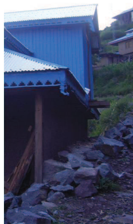
Figure 8.4 — Tower roof with more height. Source : S. Abidi
