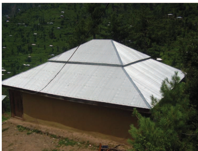
Figure 7.40 — Reconstructed house with door placed on the edge. Source : S. Abidi
