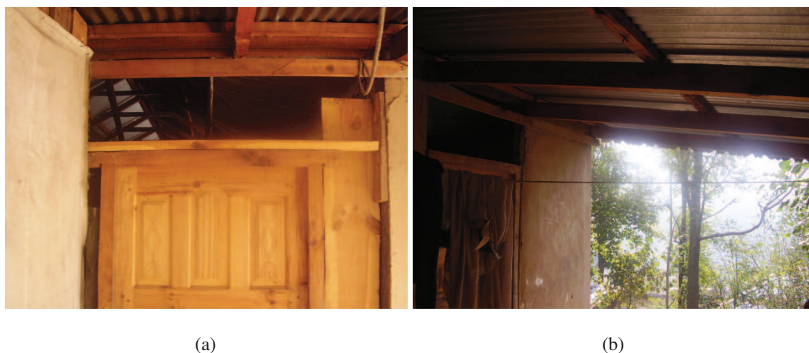
Figure 5.25 — : Opening above the doors. Source : S. Abidi.
