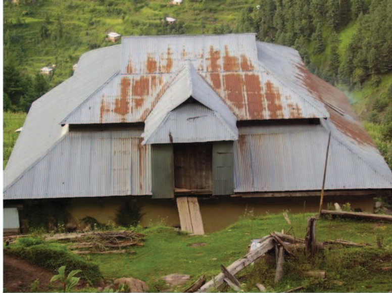
Figure 6.47 — Tower roof having a door. Source : S. Abidi
