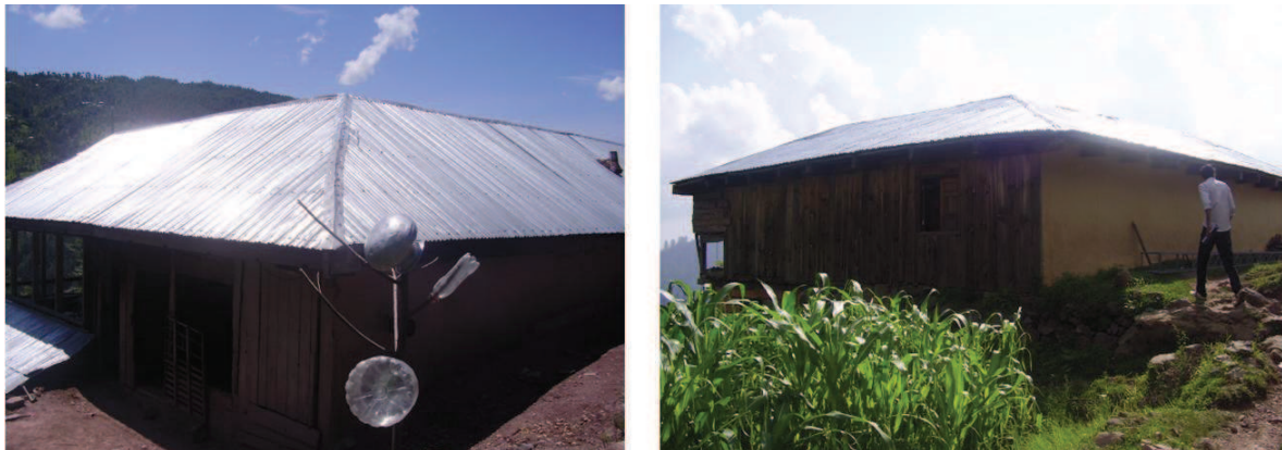
Figure 6.28 — A hip and valley roof without any break. Source : S. Abidi
