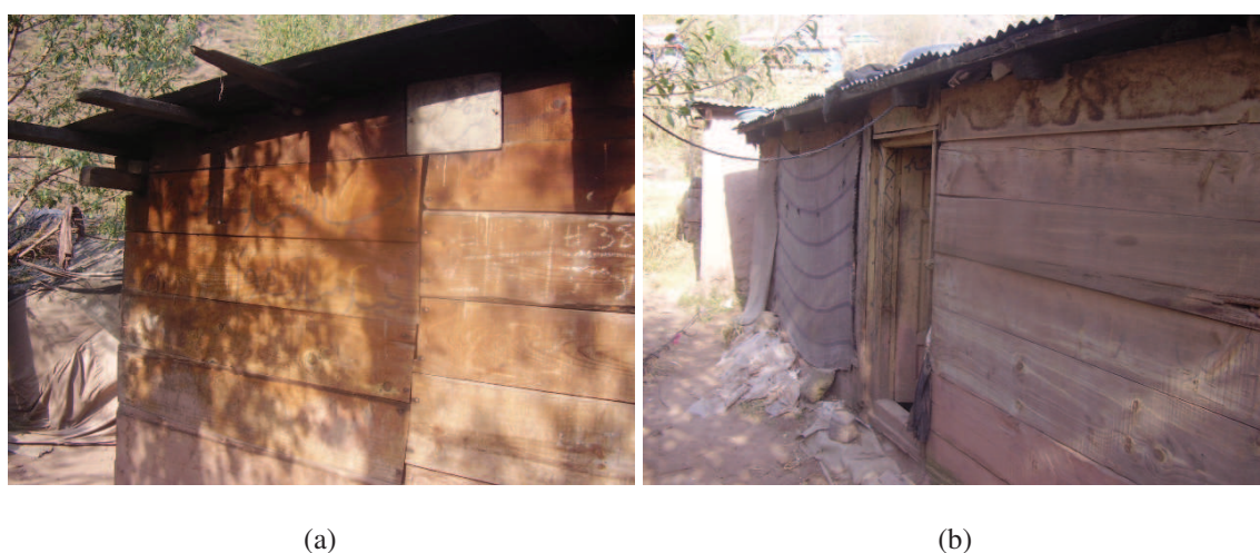
Figure 5.30 — Wooden planks are nailed on dhajji walls. source : S. Abidi
