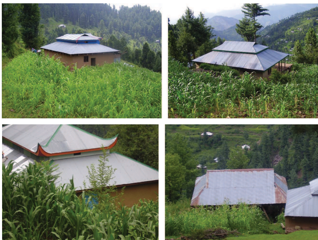
Figure 6.84 — Reconstructed houses built on agricultural land. Source : S. Abidi
