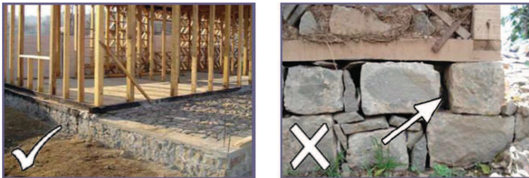
Figure 7.28 — Guidelines provided by ERRA about the gap in plinth stones. Source : [ERRA, 2008a]
