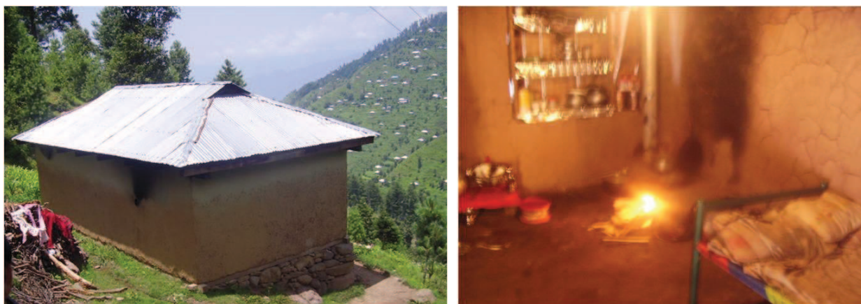
Figure 7.9 — Smoke Stains are evident on the inner and outer sides of the wall. Source : S. Abidi
