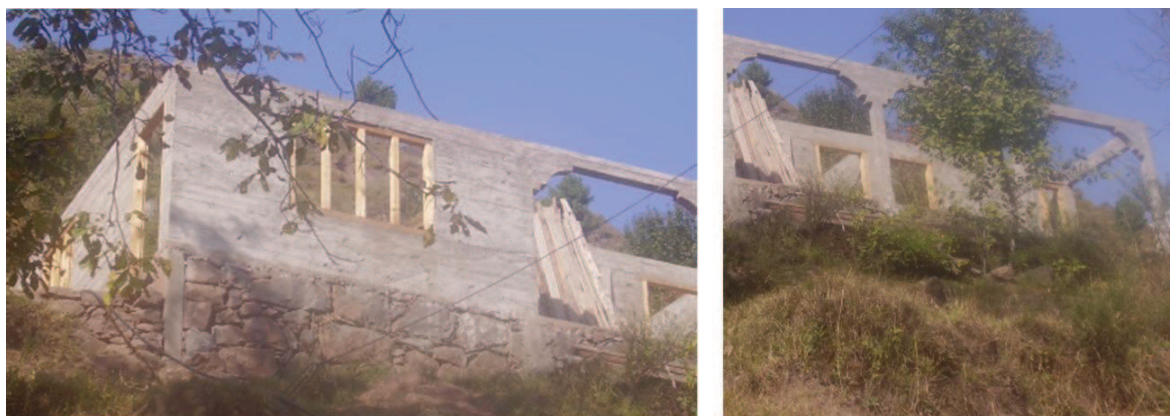
Figure 7.22 — House condition of visited vulnerable third family. Source : S. Abidi
