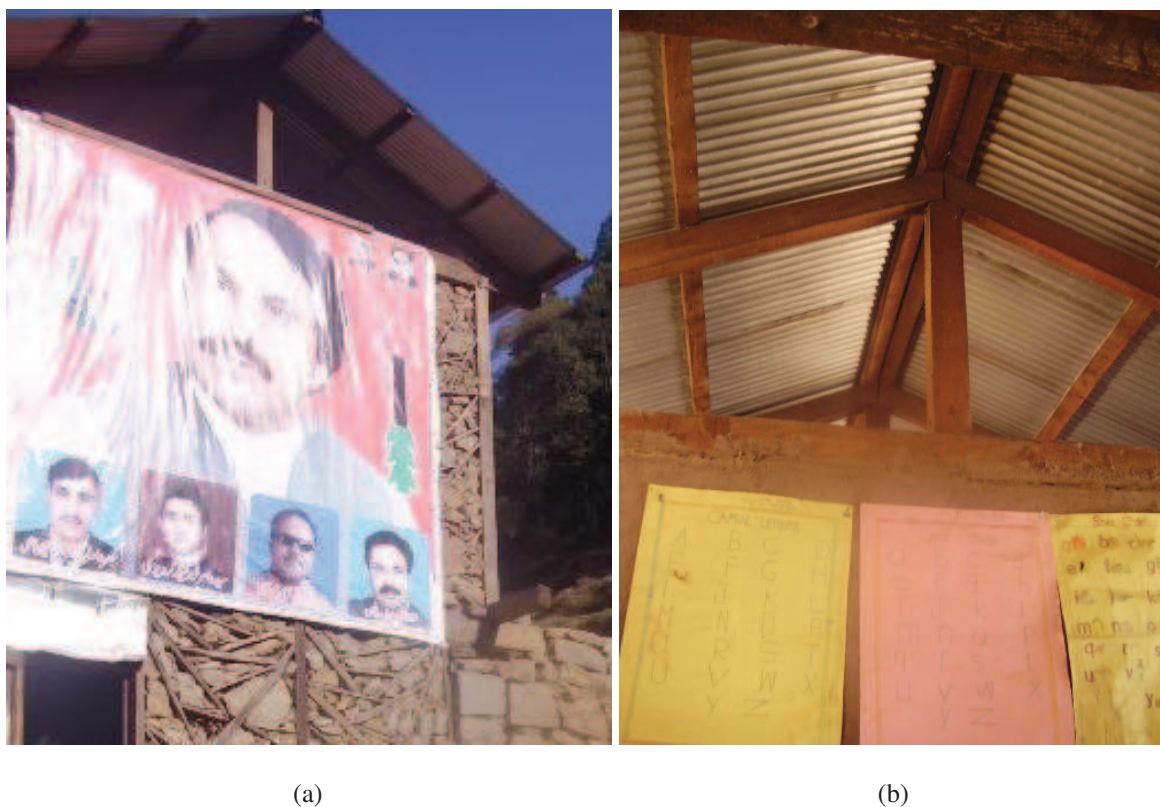
Figure 5.22 — Outside and inside views of the roof. it is not only open to the outside ; also it decreases the inner temperature because of its height. Source : S. Abidi
