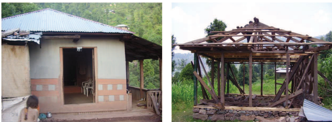
Figure 6.26 — Tower roof with hip roof without break. Source : S. Abidi
