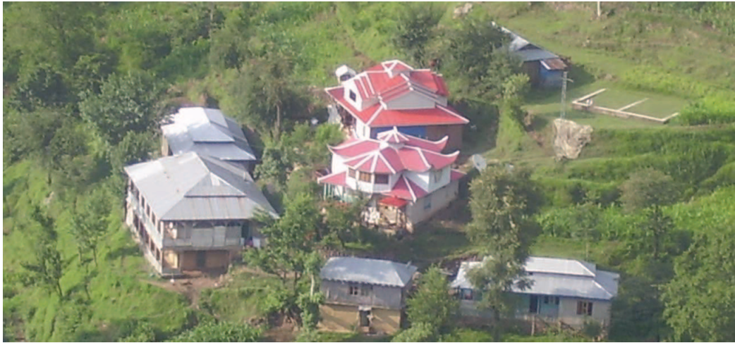
Figure 6.14 — Multiple forms of tower roof. Source : S. Abidi
