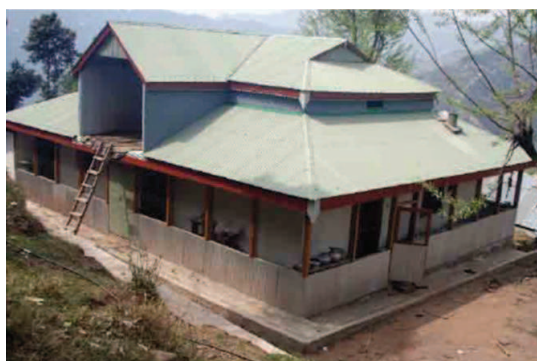
Figure 6.70 — Tower roof with accommodation. upper storey sheeted out in CGI sheets adopting light weight solution. Source : UNHABITAT Unpublished Draft, 2012
