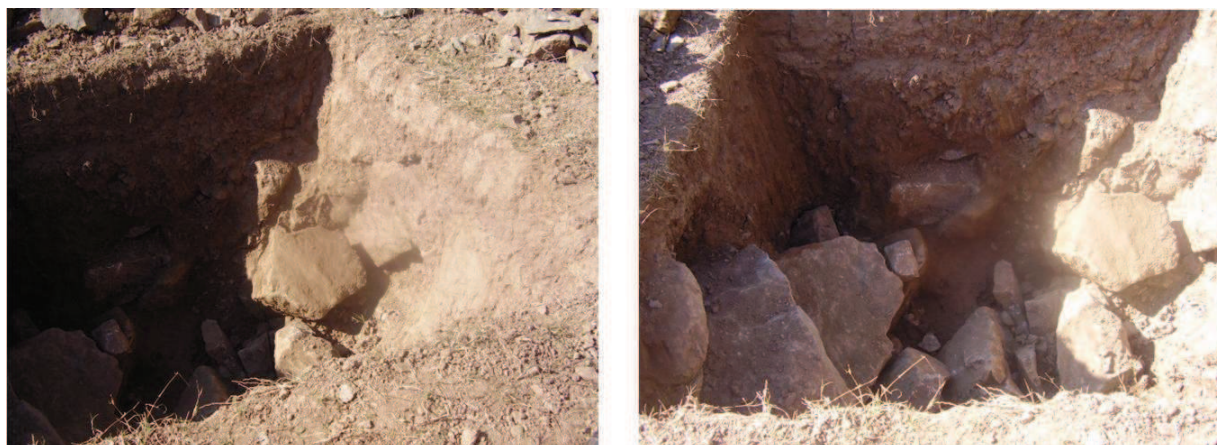
Figure 7.12 — Ditch is dug to dump the waste. Source : S. Abidi
