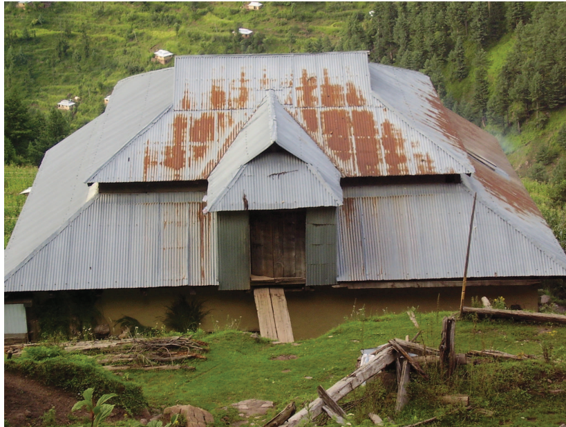
Figure 6.80 — Access from adjacent mountain, Salmia. Source : S. Abidi . Source : S. Abidi
