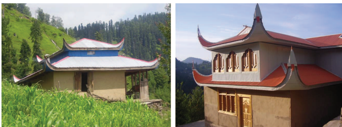
Figure 6.37 — Houses with Shangri-La roofs and prominent attic. Source : S. Abidi
