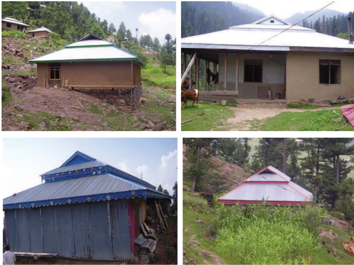
Figure 6.31 — Negligible break dutch gable roof. Source : S. Abidi
