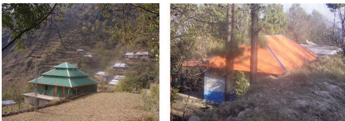
Figure 6.51 — Only few houses are found with coloured CGI sheets on the roof. Source : S. Abidi
