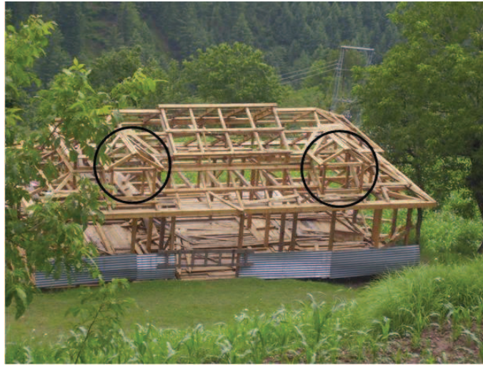
Figure 6.42 — Under-construction house having dormers. Source : S. Abidi
