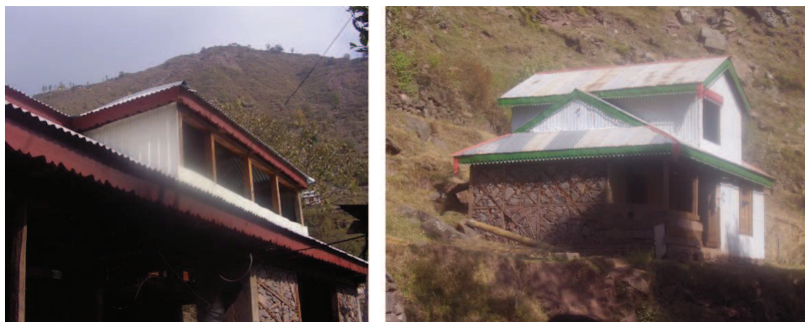
Figure 6.46 — Tower roof houses showing dhajji dewari on ground floor. the upper structure is covered with CGI sheets and is distinctly framed out of ground floor. Source : S. Abidi
