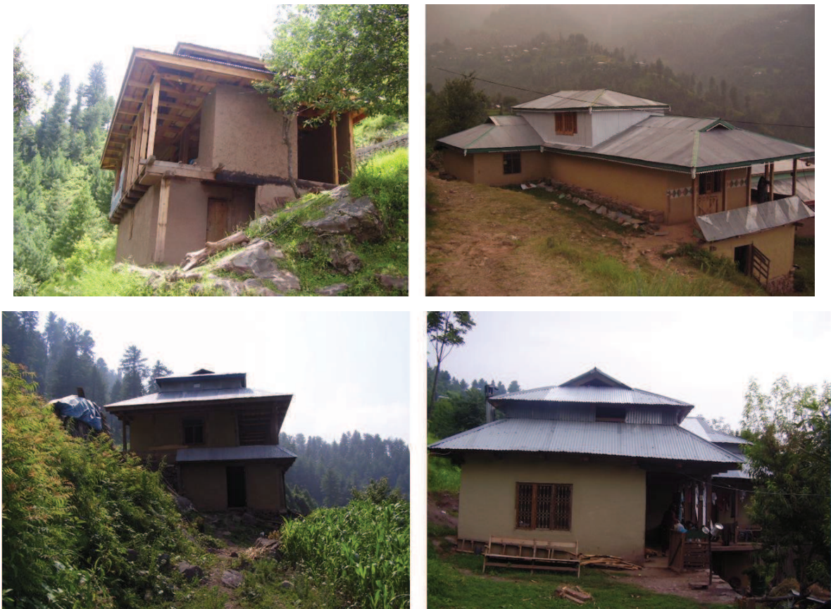
Figure 8.31 — Houses built on hazardous sites or have improper retaining wall. Source : S. Abidi
