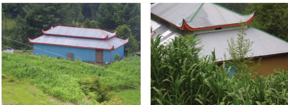
Figure 6.33 — Negligible break Shangri-La roof. Source : S. Abidi
