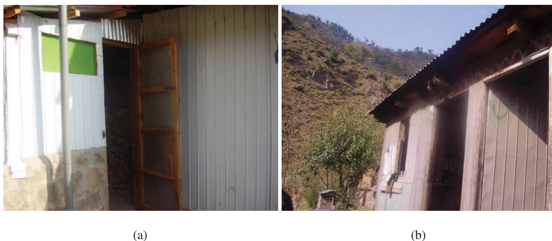
Figure 5.29 — The CGI sheets used in shelters are reused to protect walls. Source : S. Abidi.
