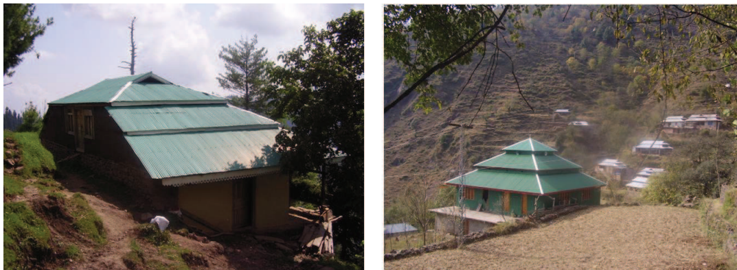
Figure 6.72 — Although negligible break in the roof is evident, the span of the roof has increased the height of attic. Source : S. Abidi
