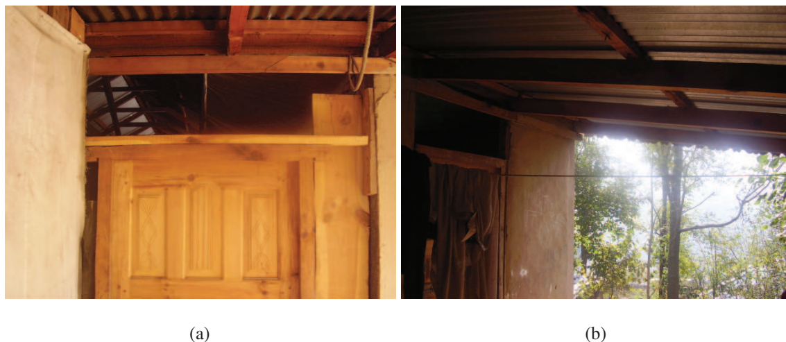
Figure 5.25 — : Opening above the doors. Source : S. Abidi.
