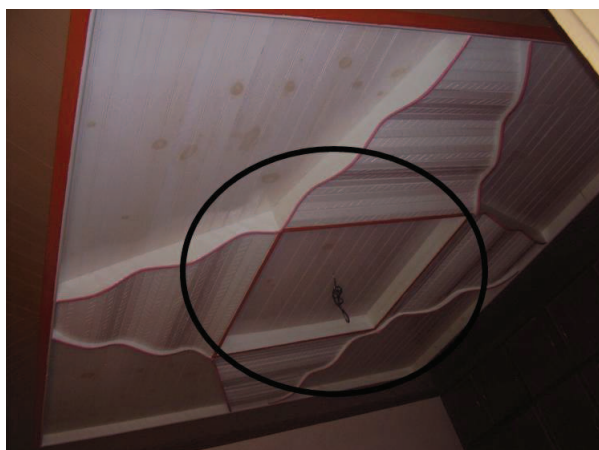
Figure 6.78 — The ceiling showing opening to enter tower roof. Source : S. Abidi
