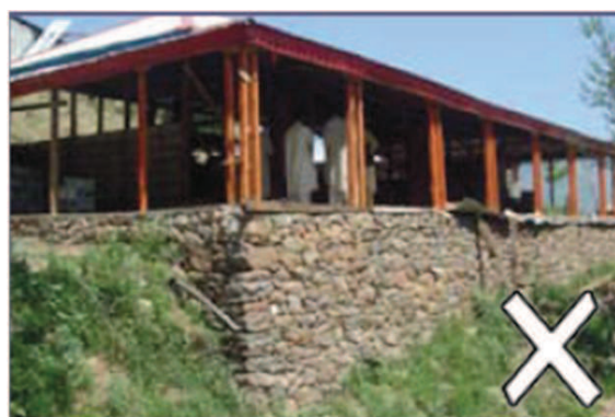
Figure 7.23 — ERRA guidelines about plinth. Source : [ERRA, 2008a]
