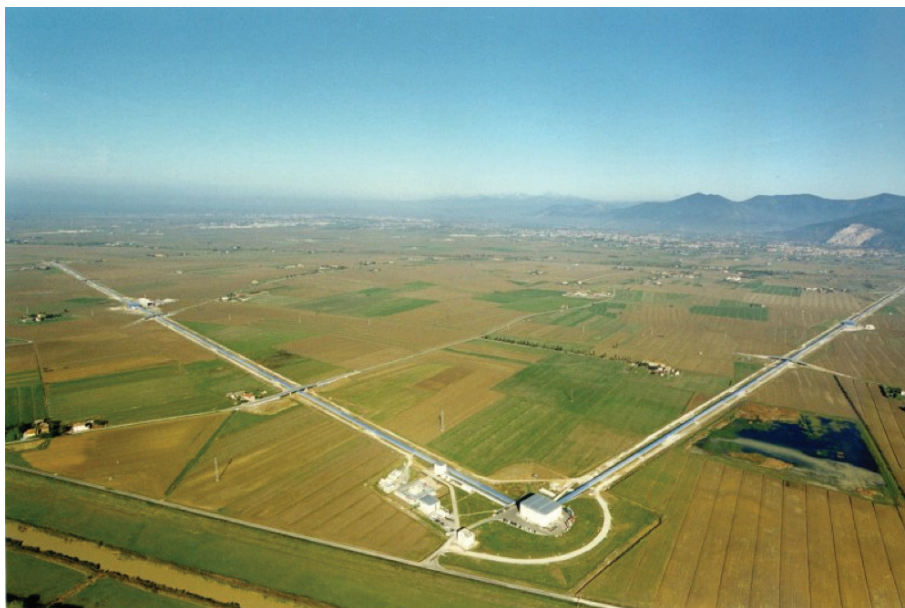
Figure 1.6: Aerial view of the gravitational wave detector Virgo.
