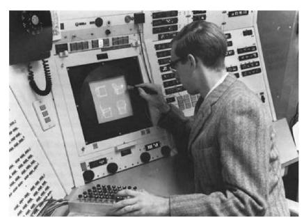
Figure 3.7: The Sketchpad system combining direct pen input on the display with physical controls for specific instruments [SUTHERLAND, 1964].
