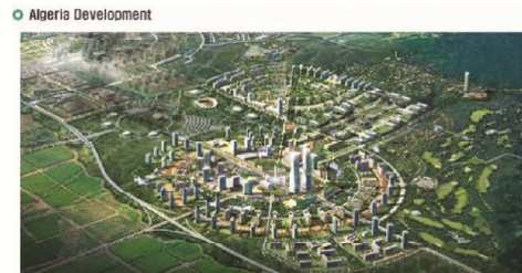
Algeria Development S.Korean firms to Build New Town In Algeria. Algeria Development Korean builders will develop 600 ha new town in the North African country of Algeria. Up to date and eco-friendly new town will have 60 thousand residents including residential, commercial, public facility and leisure complex environment. A consortium of ten South Korean builders including Bando Engineering & Construction will construct a new town in Bouin, project calls for building an ultra-modern city 30 kilometers south of Algier. Ground will be broken in first-quarter of 2008.
