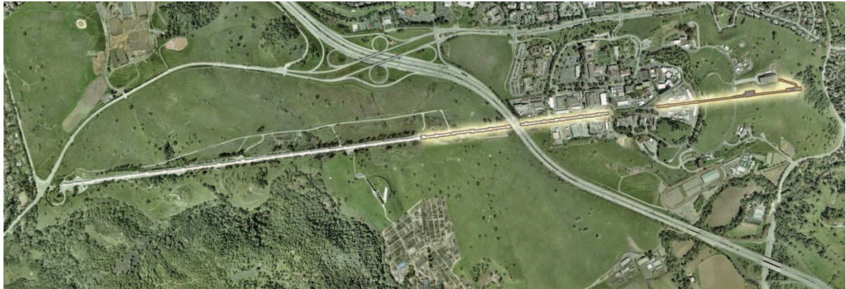
Fig 2.22 Aerial view of the LINEAC in SLAC facility.
