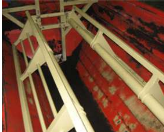
Figure 4.21 – Volets en position haute
