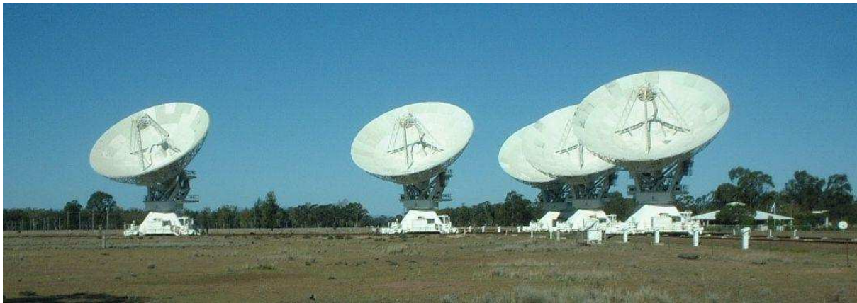
Figure 2.8: View of 5 of the 6 antennas forming the ATCA, in a compact configuration: the three antennas on the right are on the East-West tracks while the the two on the left are on the North-South track.
