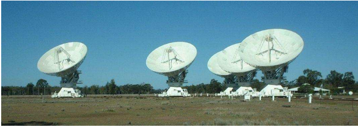
Figure 2.8: View of 5 of the 6 antennas forming the ATCA, in a compact configuration: the three antennas on the right are on the East-West tracks while the the two on the left are on the North-South track.
