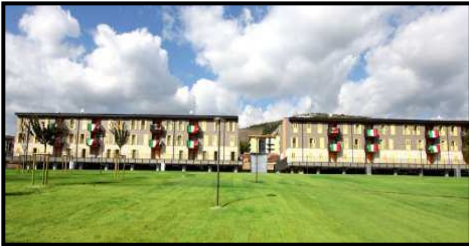
Photo 23: The new buildings in the “new” Aquila
