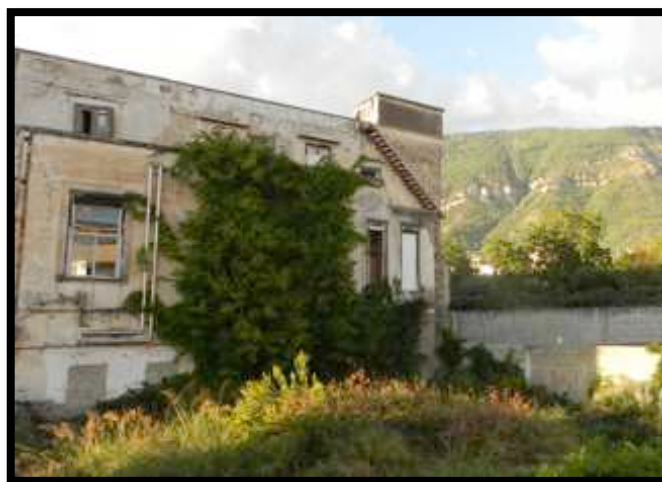
Photo 9: The Villa Malta hospital in 2012
