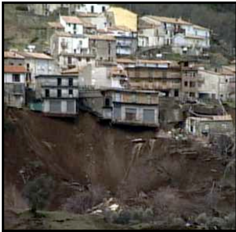
Photo 5: The Cerzeto landslide in the Cavallerizzo district
