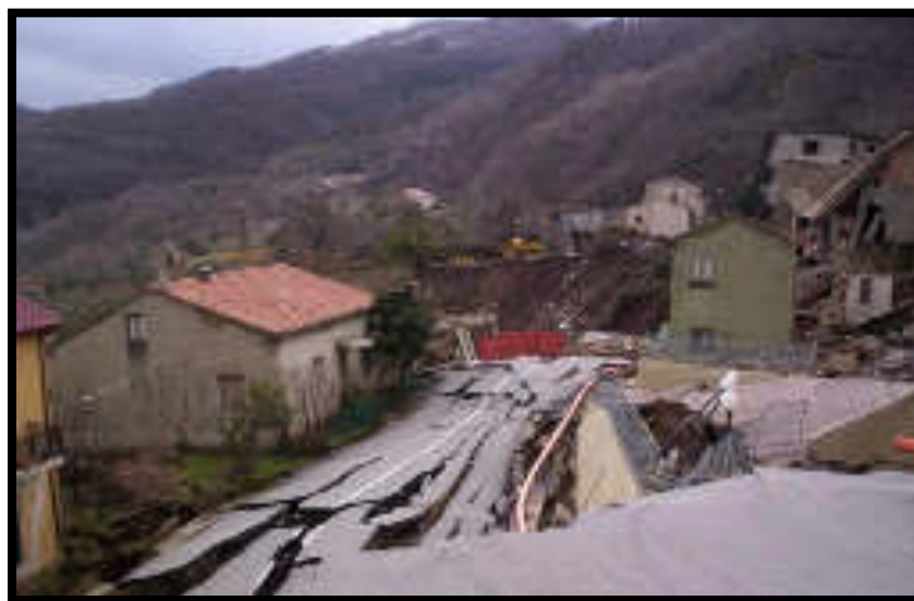
Photo 2: The Emigrants’ Road after the landslide
