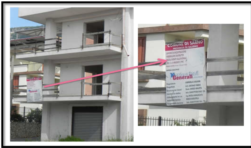
Photo 19: A building in Via Pedagnali (2012)
