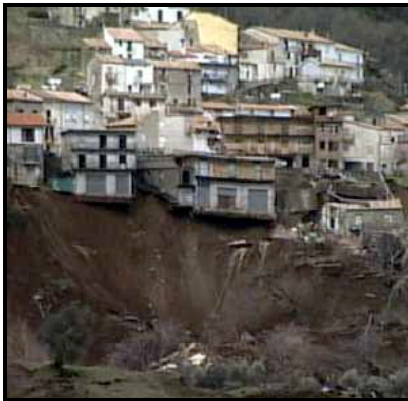
Photo 5: The Cerzeto landslide in the Cavallerizzo district
