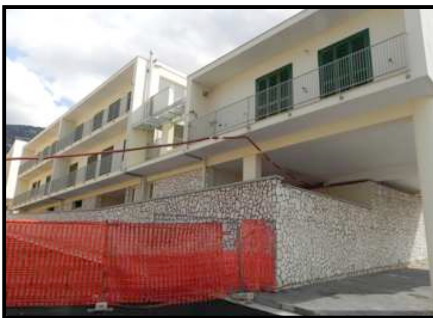
Photo 18: Housing projects in Via Episcopio, under construction
