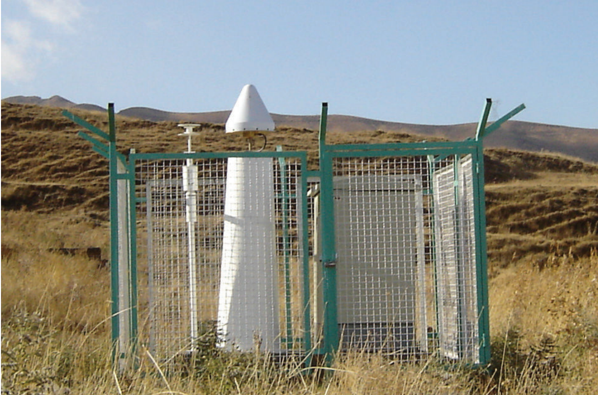
Figure 2.9 – A typical Iranian Permanent station. Each station is equipped by Ashtech Z-12 receivers, choke ring antennae and MET3A Meteorological sensor.
