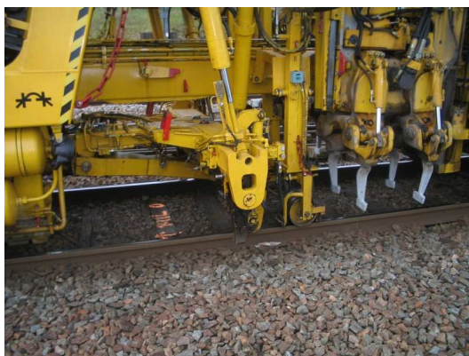
FIGURE 1.8 – Operation de bourrage.
