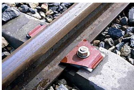
FIGURE 1.3 – Attache type nabla.
