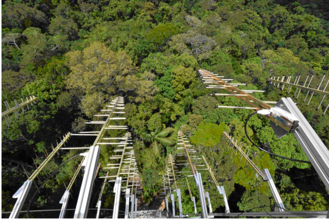
Fig. 2. Twenty antennas installed on the Guyaflux tower.
