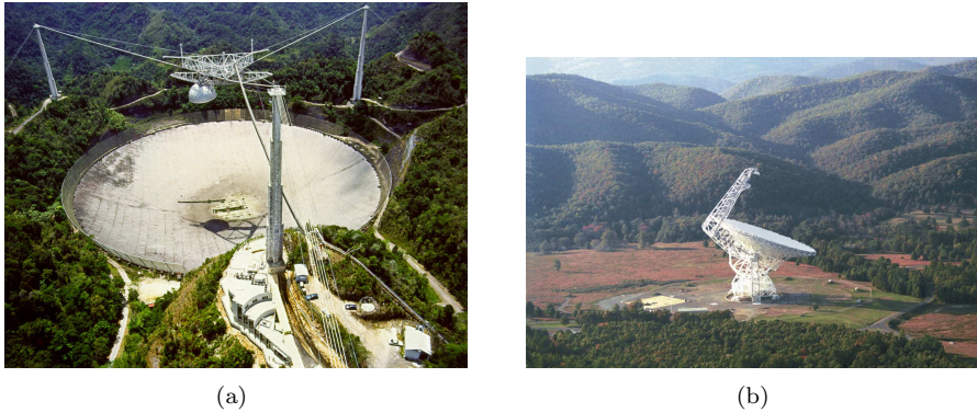
Figure 1.1: (a) Arecibo radio telescope, located in Porto Rico. 305m single dish radio telescope. (b) Green Bank telescope, located in West Virginia, USA. 100m fully steerable single dish radio telescope.
