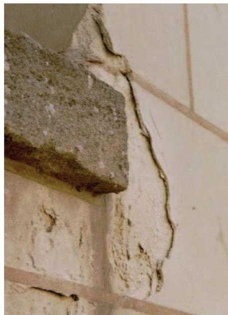
**Fig. I-16.** Stone degradation by contour scaling, Castle of Chambord, France (tuffeau limestone) (Beck, 2006).
