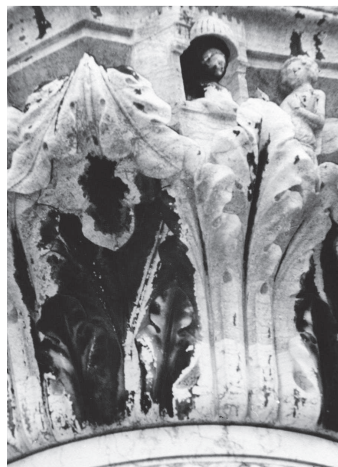
Fig. I-11. Black crust at Ducale Place in Venice, Italy (Limestone) (Maravelaki-Kalaitzaki and Biscontin, 1999).
