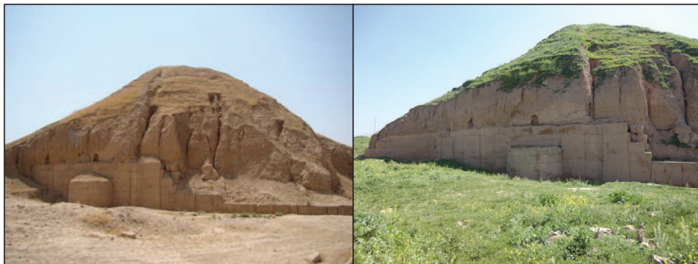
Fig. III-29. Photos showing part of Al-Ziggurat wall on its northern façade at two different periods: 27 June 2011 ( left ), and 23 March 2013 ( right ).
