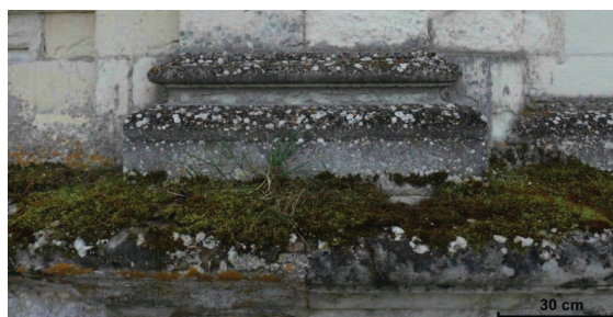
Fig. I-14. Biological colonization at the Castle of Chambord, France (tuffeau limestone) (Janvier-Badosa, 2012).
