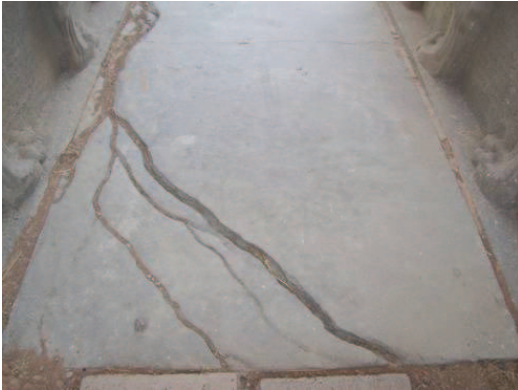
Fig. I-17. Effect of water flow in dissolving ground stone plate, Al-Nimrud monument, Iraq (marble).
