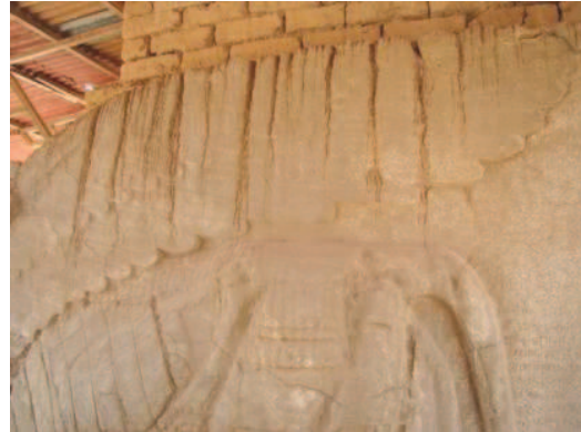
Fig. I-18. Effect of water flow in dissolving the winged sculpture, Al-Nimrud monument, Iraq (marble).
