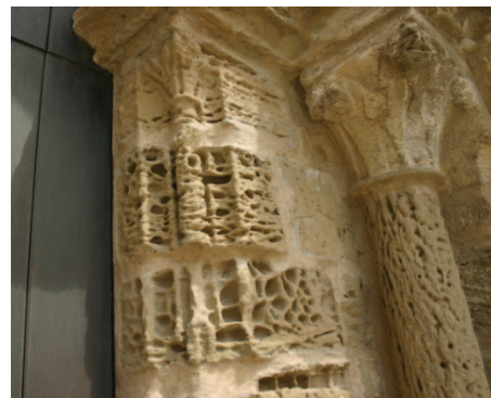
Fig I-6. Honeycomb, St. Leonardo's church, Portugal (Sandstone) (Ludovico-Marques et al., 2012).
