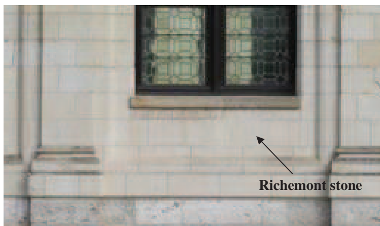
Fig. II-4. Richemont stone on the wall of the Castle of Chambord used in the restoration work in 1955, (Janvier-Badosa, 2012).
