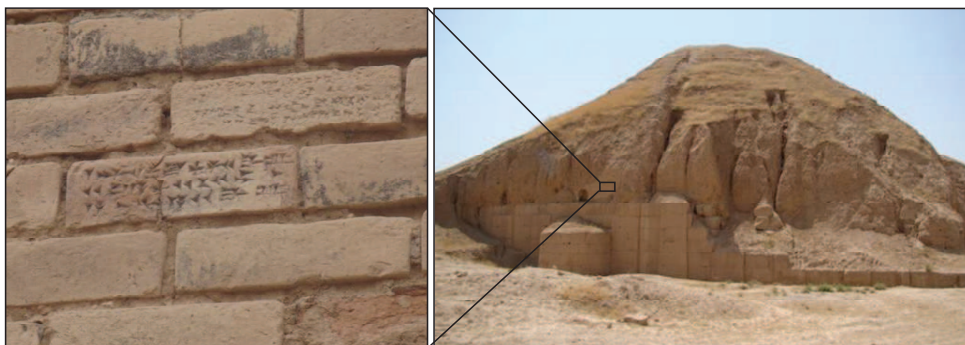
Fig. III-15. General view of Al-Ziggurat showing the north, the west walls and the brick-clay layer above the wall ( right ); the Cuneiform script on the clay-brick ( left ).
