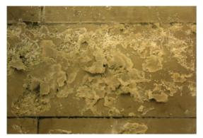
**Fig. I-5.** Efflorescence, Crypt of the Cathedral of Cádiz, Spain (Limestone) (Vázquez et al., 2011).
