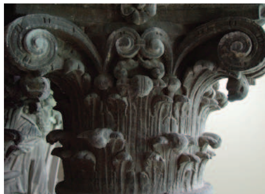
Fig. I-12. Black crust at cathedral of Granada, Portada del perdon, Spine (limestone) (Maravelaki-Kalaitzaki and Biscontin, 1999).
