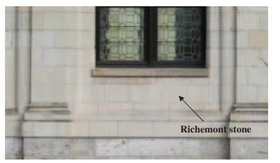
**Fig. II-4.** Richemont stone on the wall of the Castle of Chambord used in the restoration work in 1955, (Janvier-Badosa, 2012).
