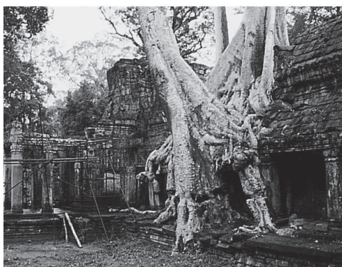
Fig. I-13. Roots of a tree growing on the monument, Ta Prohm-Angkor monument, Cambodia (Uchida et al., 1999).
