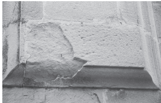
Fig. I-15. Stone degradation by flaking, church of San Mateo, Spain (Sandstone) (Sebastián et al., 2008).
