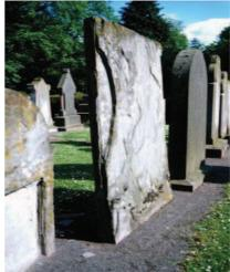
**Fig. I-2.** Delamination of a gravestone possibly by frost action, Cathedral Graveyard, Scotland (Sandstone). (ICOMOS-ISCS 2008).
