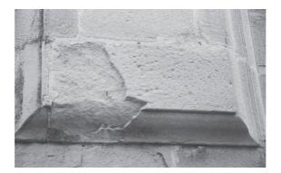
**Fig. I-15.** Stone degradation by flaking, church of San Mateo, Spain (Sandstone) (Sebastián et al., 2008).
