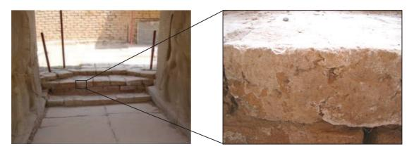
**Fig. I-7.** Granular disintegration by salt weathering, Al-Nimrud monument, Iraq (Limestone).
