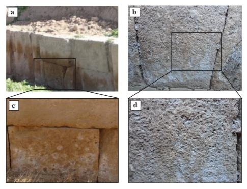
**Fig. III-16.** Field photographs showing: (a) and (b) the degraded stones on Al-Ziggurat wall; (c) and (d) details of salt weathering showing the decay patterns: granular disintegration, powdering and sanding.
