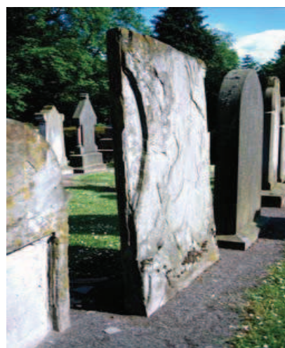
Fig. I-2. Delamination of a gravestone possibly by frost action, Cathedral Graveyard, Scotland (Sandstone). (ICOMOS-ISCS 2008).
