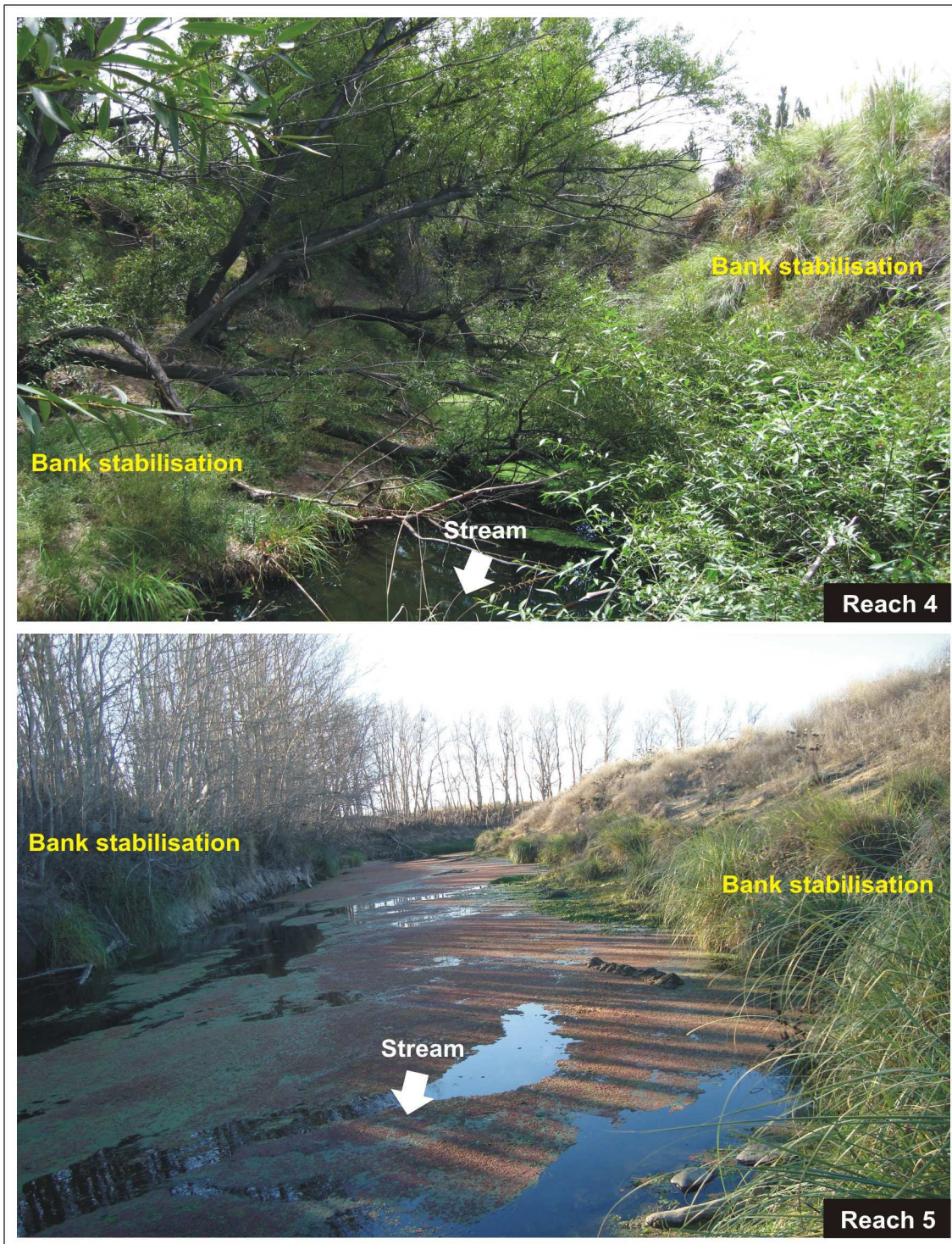
Figure 5.16: Evidence of channel stabilisation within the river downstream. Photographs were taken on river reaches located about 1 km (Reach 4) and 5 km (Reach 5) downstream from the dam closure.
