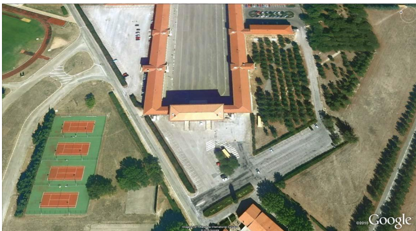
Figure 2.7: Main building of Air Force Base area.
