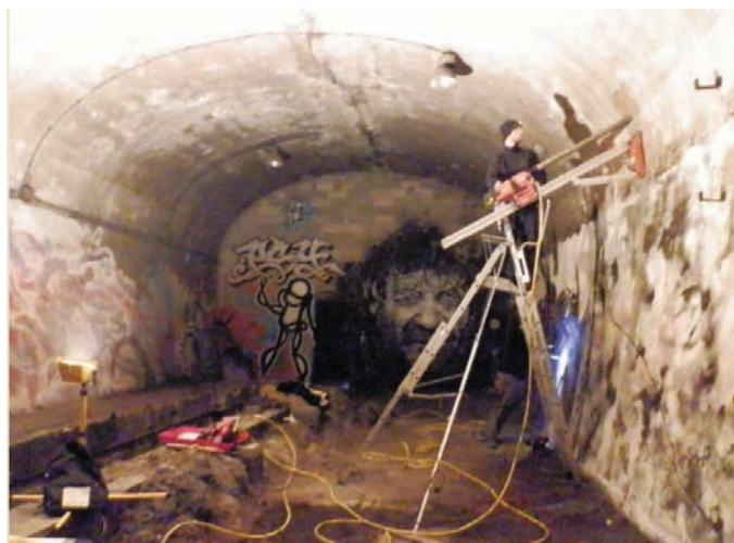
Figure 5-5 Tunnel station Porte de Vanves
