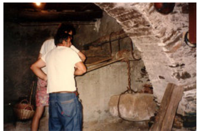
Figure 41: pressurage/Photo Eddy Retali
